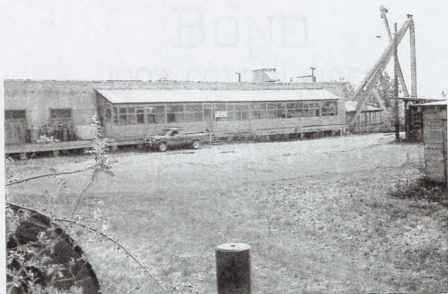
Figure 17. Warehouse 1, looking across the warehouse yard from the north. 1992 photo by the author.
