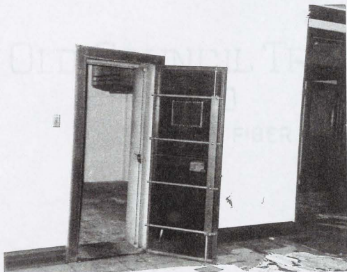
Figure 14. Office Building, 1992. Door to second floor vault. Photo by the author.
