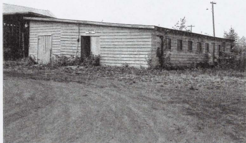
Figure 26. Warehouse 6 from the east, with Warehouse 5 attached at the extreme right. Part of one of the steel racks is visible to the left; the warehouse yard is in the foreground. 1992 photo by the author.
