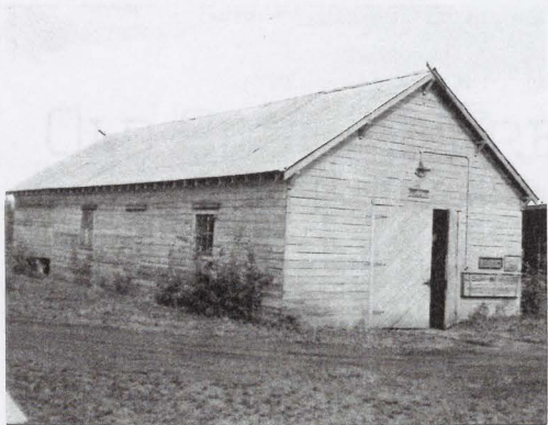
Figure 24. Warehouse 3 from the south. The rack to the right of the doors stored fire hose. 1992 photo by the author.
