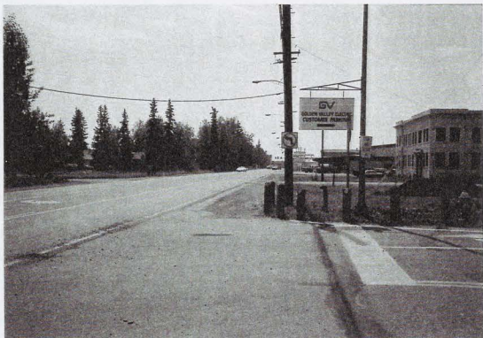
Figure 6. Illinois Street looking south towards downtown. The F.E. Office Building is on the right; F.E. Residences 7-10 are in the trees in the left center. July 1993 photo by the author.
