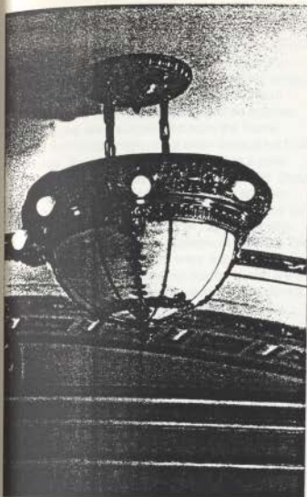
Figure 177. Lobby alcove luminaire
