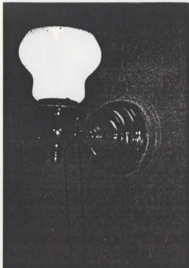
Figure 19. Bathroom wall bracket fixture
