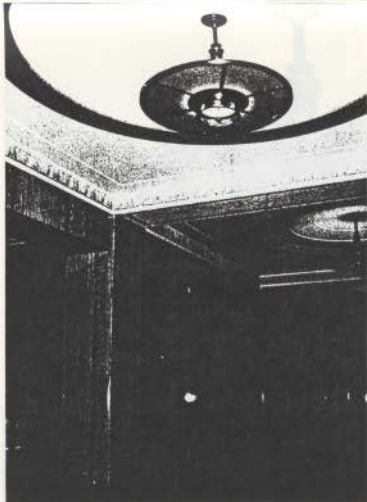
Figure 1. 2 First Floor Lobby
