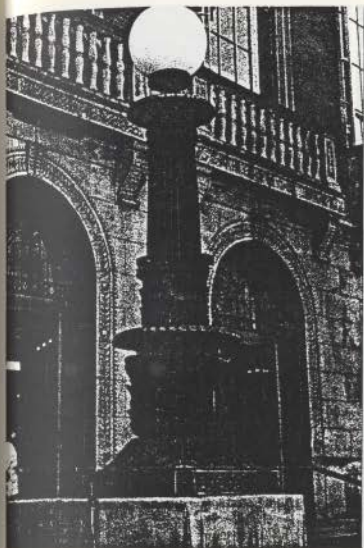
Figure 163. Portland Central Library entrance lantern
