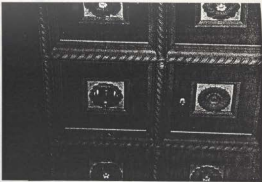
Figure 23. Detail of the downlight installation
