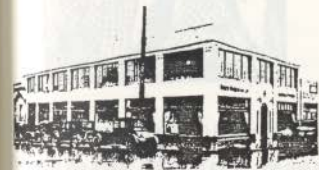
Figure 155. The English-Baker shop of the 1920's on Morrison Street, later replaced by the freeway
