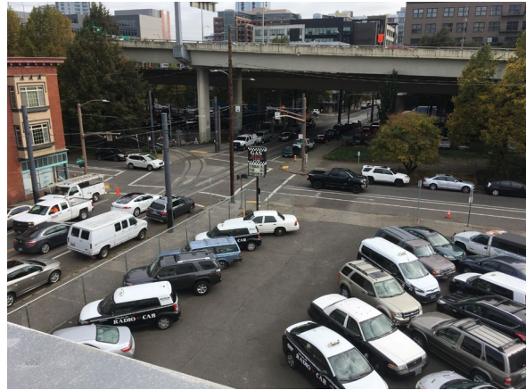
Figure 4: Exterior pollutant sources include an adjacent parking lot and the I-405. Source: (Elise Braun 2019)
