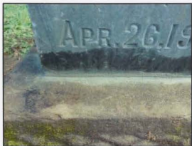
Detail of fresh mortar joint
