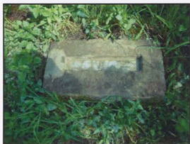
Base after mortar removal
