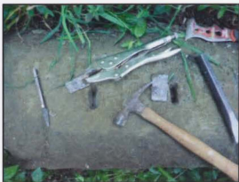
Removal of cast iron pins
