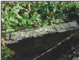
Detail of epoxy 'dollops'
