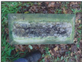
Detail of failed bonding materials on base
