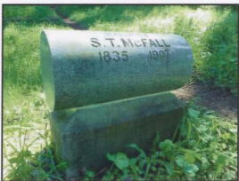
Detail of failed bonding materials on base
