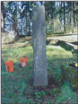
West (rear) façade pre-treatment
