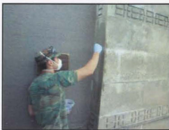
David Espinosa testing Lime-Solv on efflorescence
