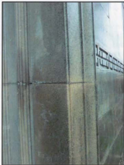
Efflorescence post-treatment
