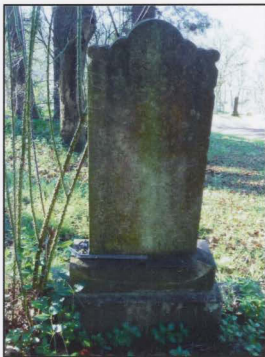
East face of Osburn marker pre-treatment. Note middle element repair.
