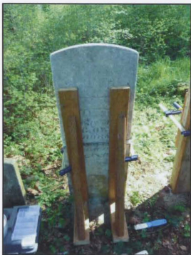
Lumber supports in place during curing
