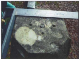
Detail of missing element
