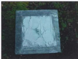
(Above) Lower marble element after mortar removal (Below) New mortar application
