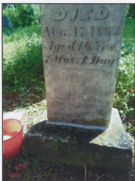
Mortar bed detail
