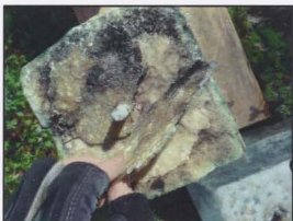
Removal of epoxy at fracture
