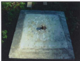
(Above) Lower marble element after mortar removal (Below) New mortar application
