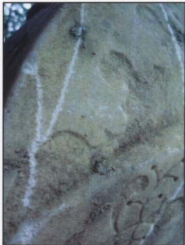
Detail of gouging, and natural accretions
