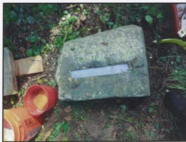
Recessed slot with mortar bed prepared
