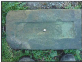
Recessed slot clear of mortar and cleaned
