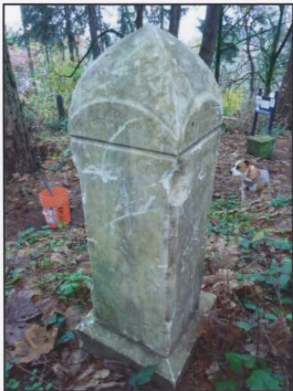
South corner of marker pre-treatment. Note material loss and conservation dog
