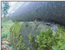
Detail of caulked joint
