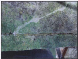
Detail of yellow epoxy and white mortar
