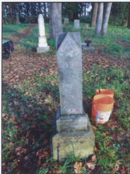
West face post-treatment
