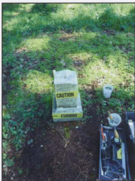
(Above) Curing of mortar joint
