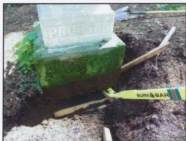
Leveling of the Packard marker
