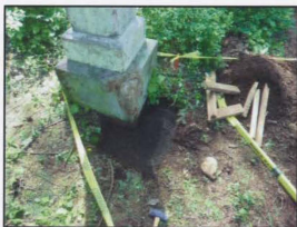
(Above) Gravel tamping and associated tools
