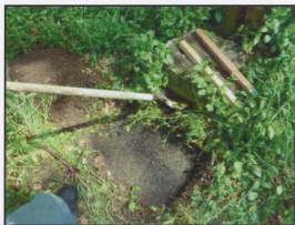
Gravel bed set for base relocation
