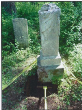
Pry-bar in use as gravel infill is inserted
