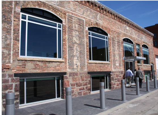
Figure 1. Exterior of the new DesignWest studio, located in an 1890s-era steam-boiler plant. Photo: Carol Faber.
