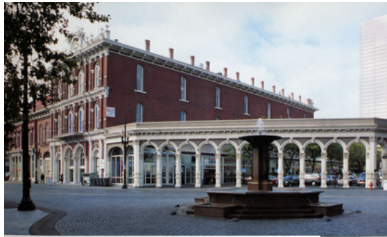
Figure 3. 1872 New Market Theater, with the re-installed North Wing cast iron arcade. Photo: Sarah Steen.
