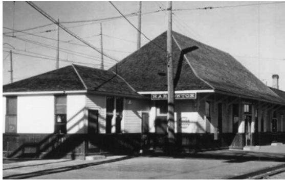
Figure 4. The residents of Harlowtown managed to preserve the Harlowtown Milwaukee Depot (above). Photo: Harlowton Chamber of Commerce www.harlowtonchamber.com/milwaukeeerr.html
