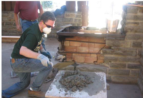
Figure 1. Tim Askin, an incoming historic preservation graduate student, repairing the central triple cook stove in the kitchen shelter. Photo: Abby Glanville.
