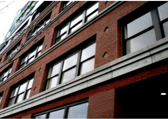
Figure 4. The White Stag Block, historically known as the Hirsch-Wiez Block, is an excellent example of the direction the University of Oregon is taking to lessen its ecological footprint. Photo: Jolyn Overton
