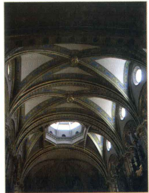
Top: buttresses and oculus windows of the side elevation. Right: intricate rib vaults of the interior. Photos courtesy of Natalie Perrin.
