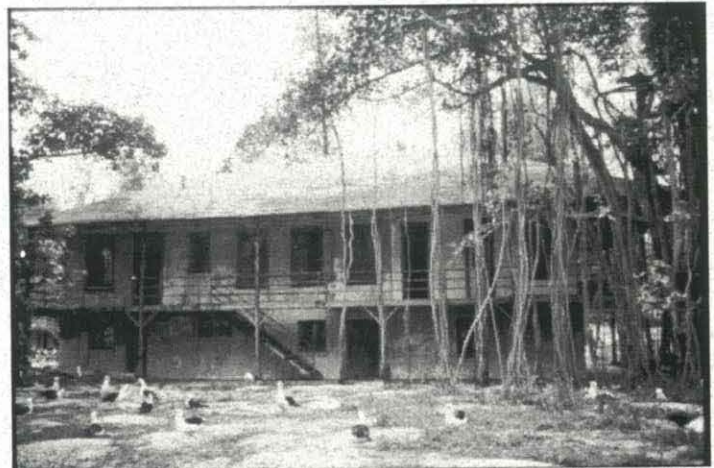
One of the Commercial Pacific Cable Company buildings on Midway. Photo by the author.
