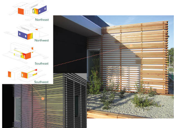
Figure 5. INhouse climatically responsive redwood screen design. Solar Cal Poly, 2015
