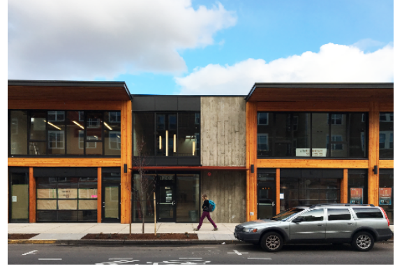
New retail and office building on Willamette St. Photo by: Paige Portwood
