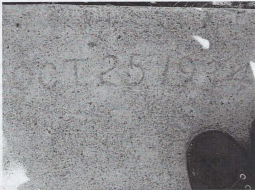
Figure 9. Blue Ridge Lookout, California. Foundation Construction Date. (Photo by Author, 2009).
