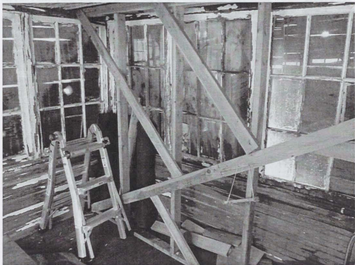
Figure 22. Olallie Mountain Lookout interior bracing work, (photo by author, October 20, 2012).
