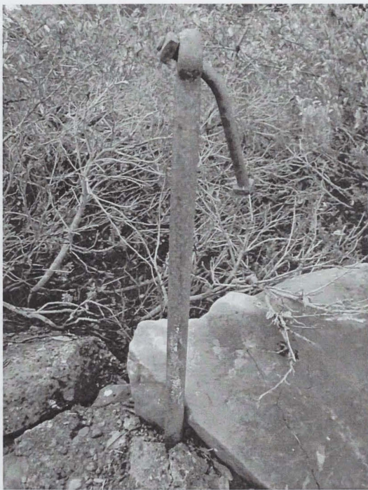
Figure 27. Steel guy wire anchor at Frissell Point Lookout site (photo by author, November 3, 2012).
