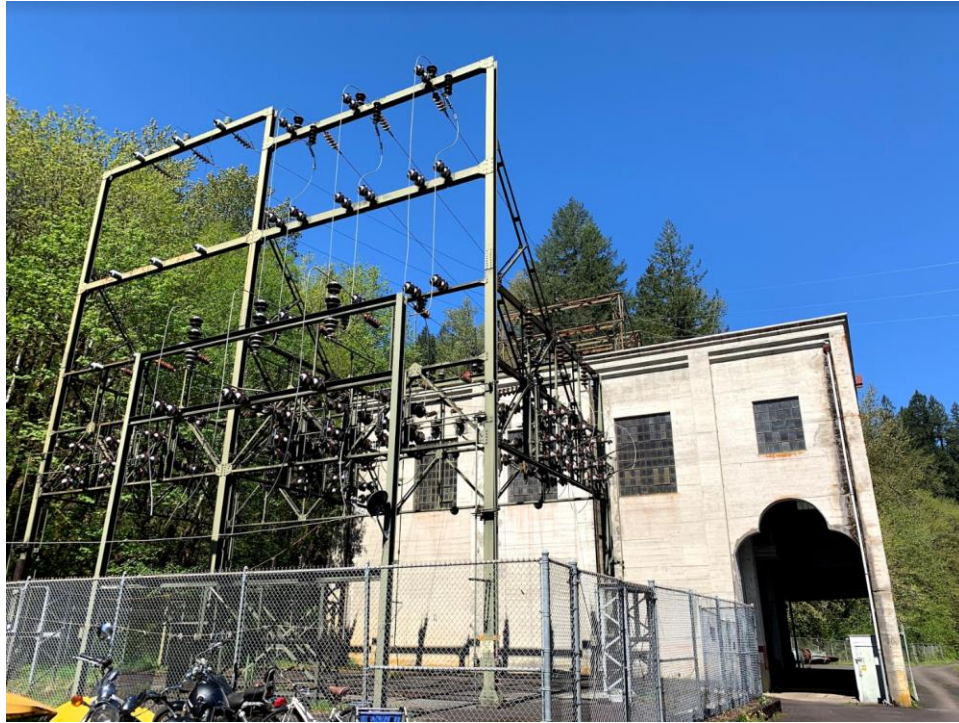
Figure C-21 Exterior of Bull Run transmission building. Source, author.
