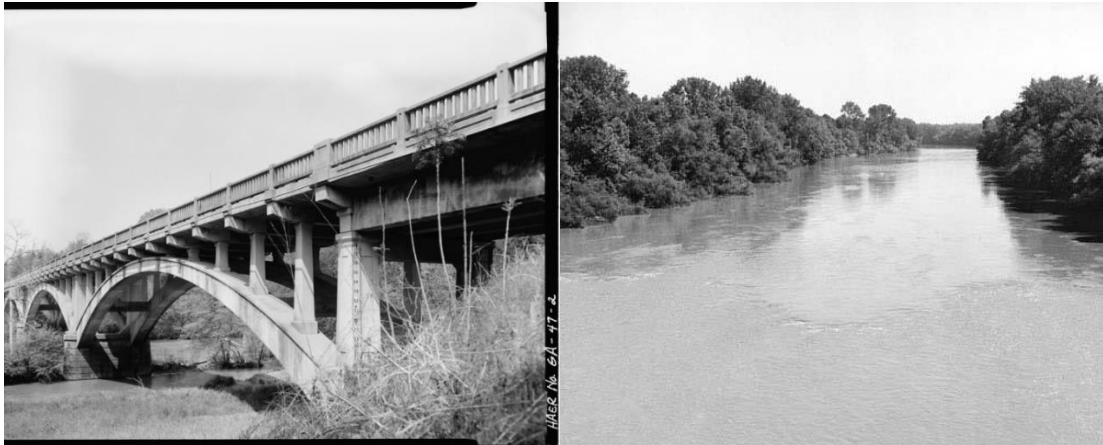
Figure 6.1 (left) Historic Broad River Bridge, constructed 1935, decommissioned 2003. Source: Library of Congress. Figure 6.2 (right) Historic Fish Weir on Broad River. Source: South Carolina Department of Archives and History.
