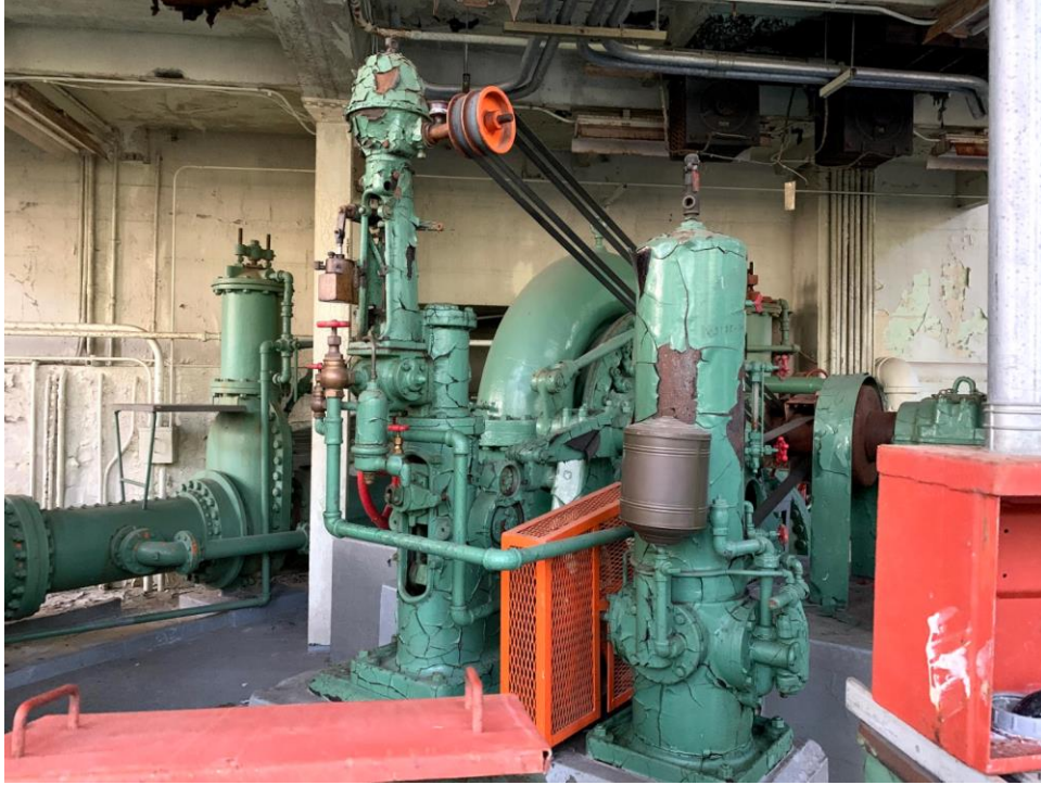
Figure C-35 Mechanics in the Bull Run Powerhouse. Source, author.
