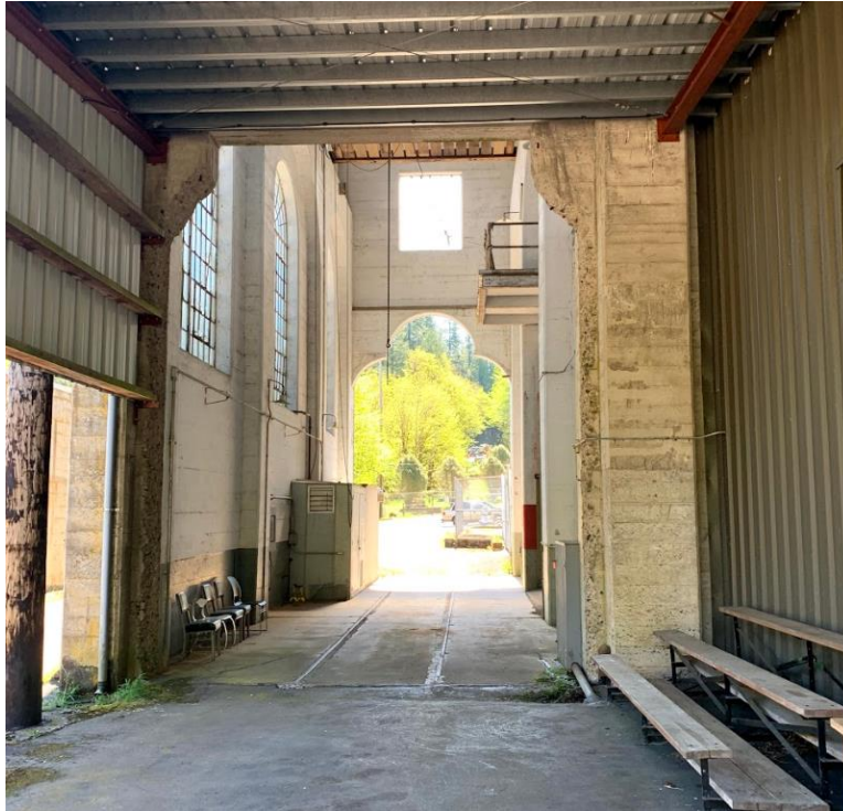
Figure C-31 Final remaining section of train tracks at Bull Run Hydroelectric Site, located within the Bull Run Transmission Building. Source, author.
