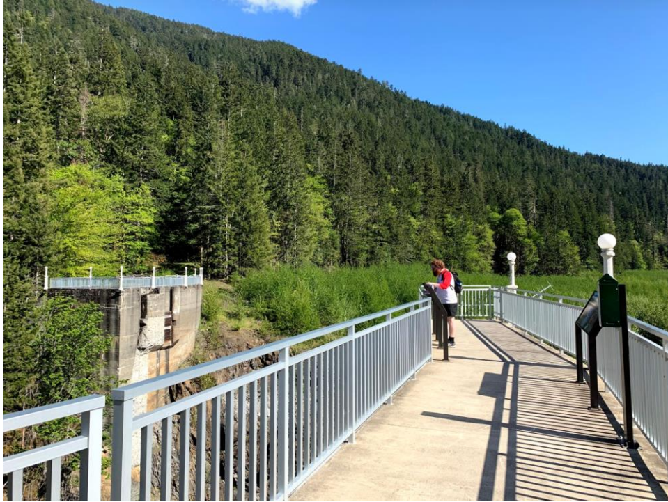
Figure C-66 Glines Canyon Spillway Overlook. Source, author.
