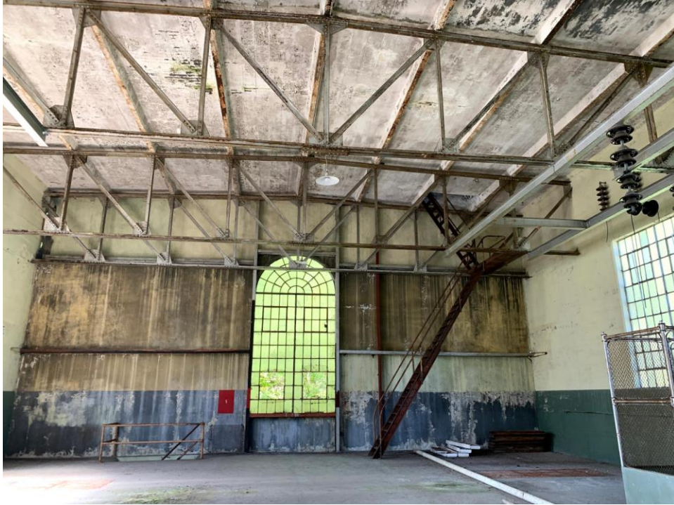
Figure C-29 Bull Run Transmission Building second-story interior. Source, author.
