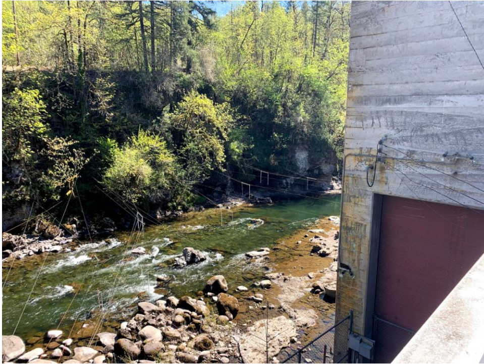
Figure C-33 Bull Run River and the Bull Run Powerhouse. Source, author.
