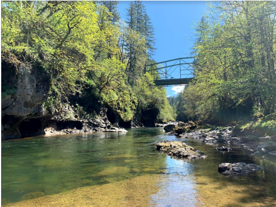
Figure C-39 View of the Bull Run River upstream from the Powerhouse.
