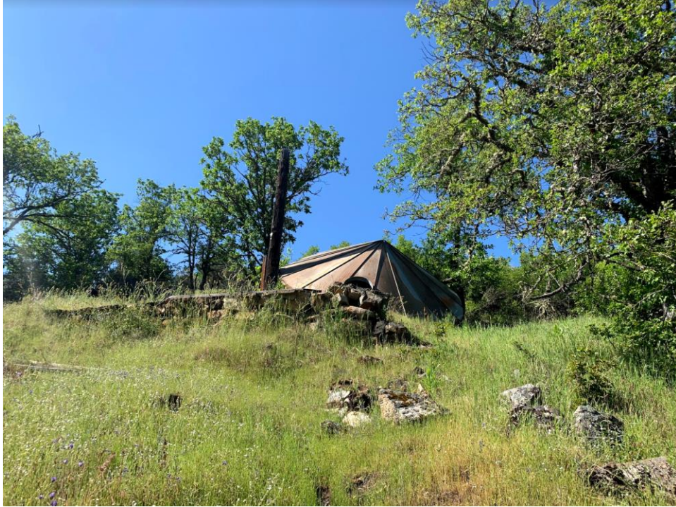
Figure C-19 Original Gold Way water tank. Source, author.
