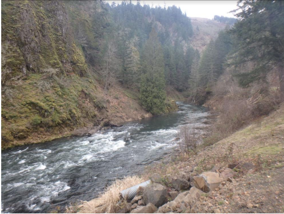
Figure C-5 View upstream of the White Salmon River from the Condit Powerhouse. Source, author.
