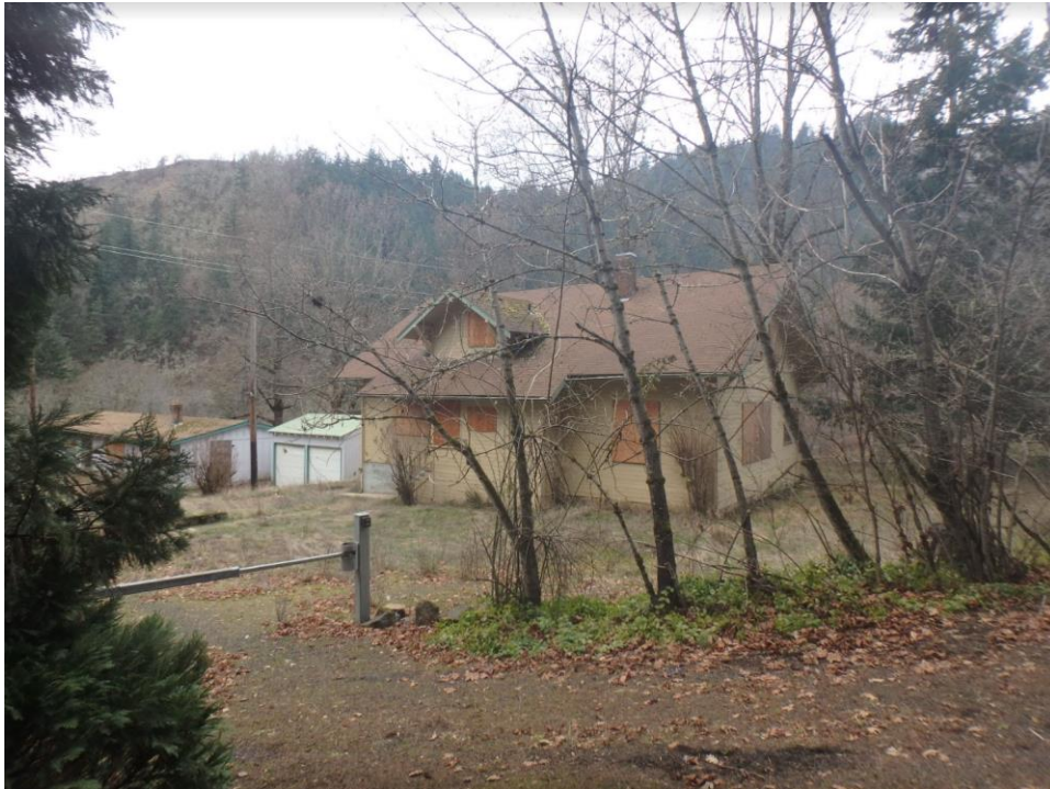
Figure C-1 Boarded up buildings at the Condit Hydroelectric Site. Source, author.
