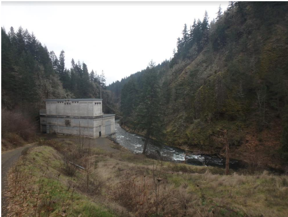
Figure C-3 Rear of Condit Powerhouse and gravel access road. Source, author.
