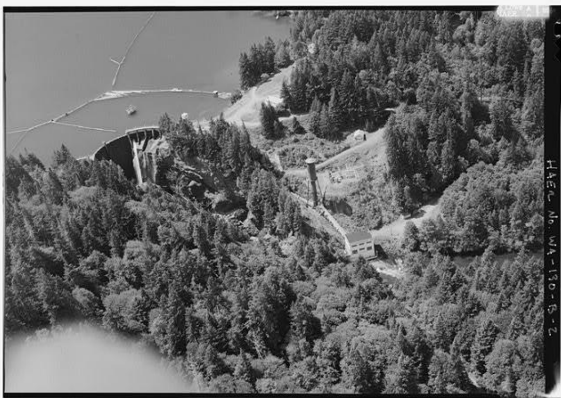
Figure 7.12 The Glines Canyon Dam, Powerhouse, and reservoir, 1995. Source: The Library of Congress.
