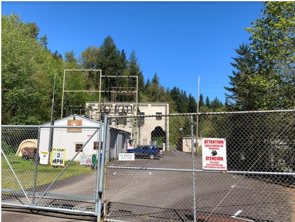
Figure C-20 Entrance to Bull Run Hydroelectric project. Source, author.
