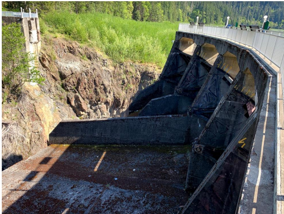
Figure C-57 Glines Canyon Spillway Overlook, view of preserved spillway. Source, author.
