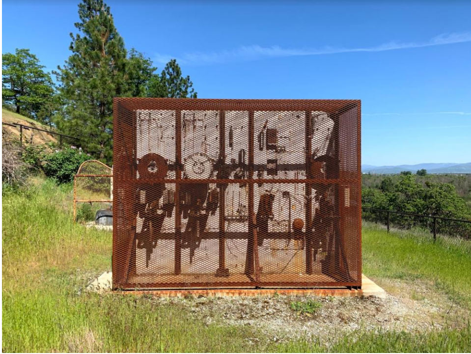
Figure C-17 Gold Ray Powerhouse original control panel. Source, author.
