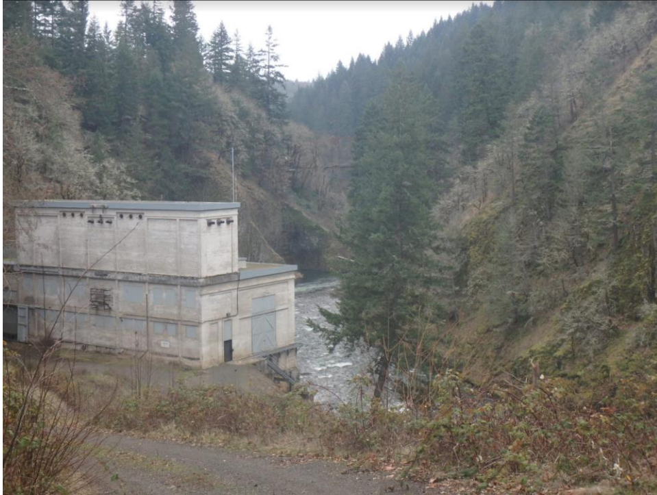
Figure C-2 Rear elevation of the Condit Powerhouse located on the White Salmon River. Source, author
