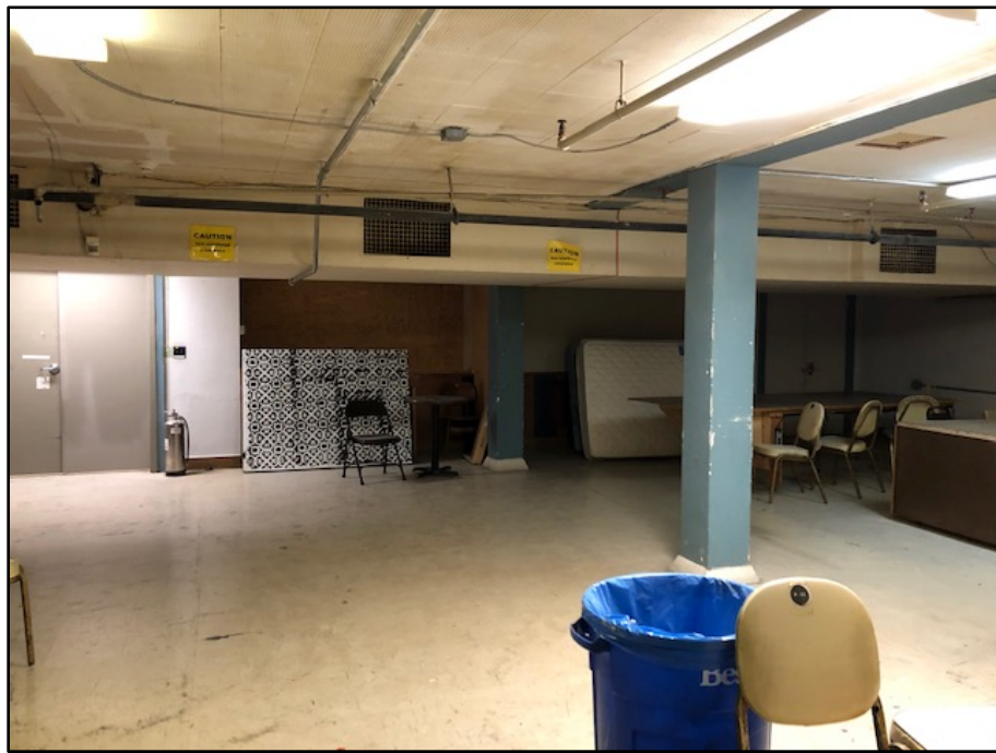
Figure 37. Backstorage in basement of the building. Photo by author.
