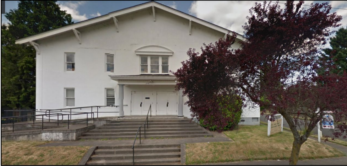
Figure 44. Vacant building for sale in state of deferred maintenance. Credit, Google Maps (2011).
