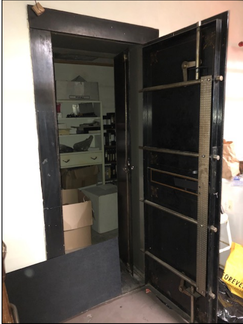
Figure 38. Vault located in the basement of the building. Photo by author.
