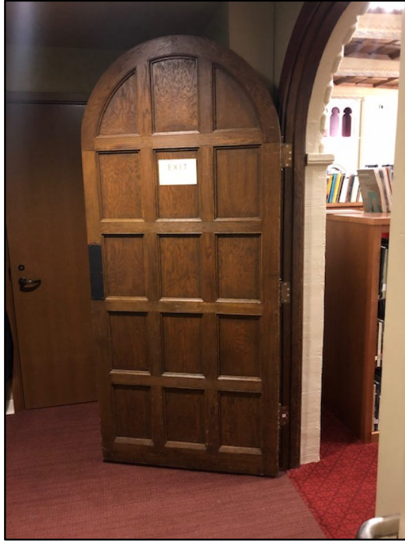
Figure 29. Arched doorway in Research library. Photo by author.
