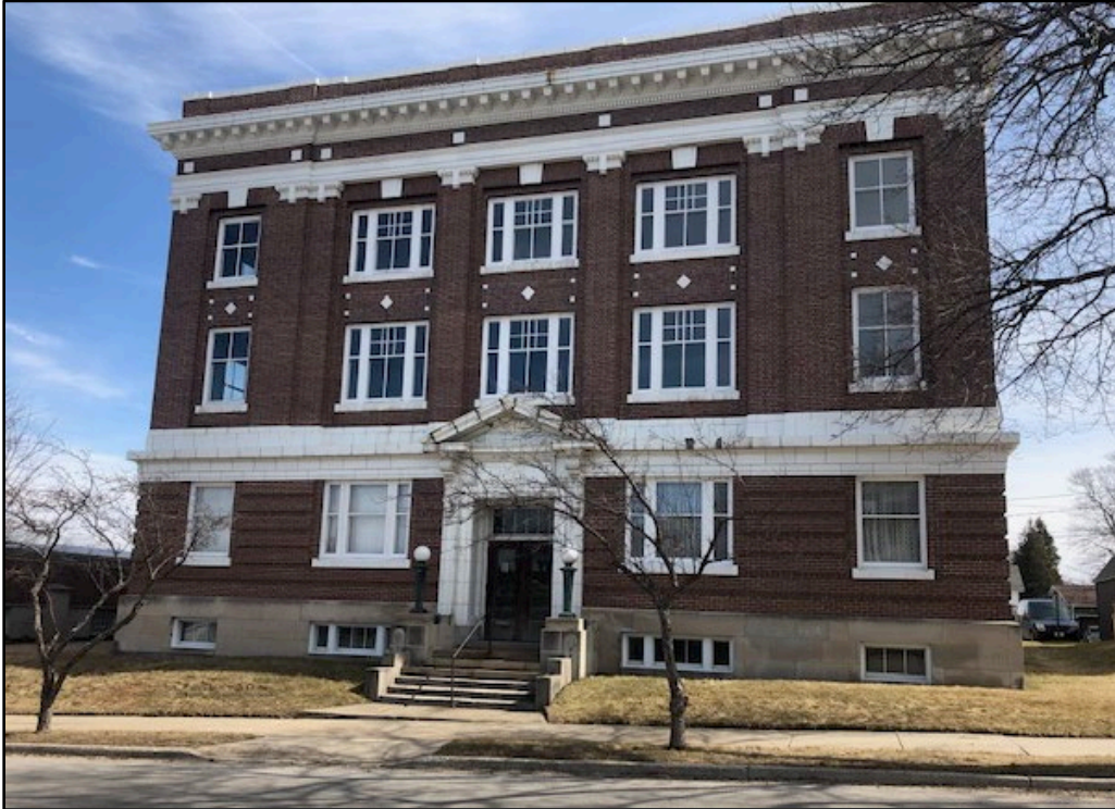
Figure 7. Former Manistee Masonic Lodge, Manistee, MI awaits new use. Photo by author.
