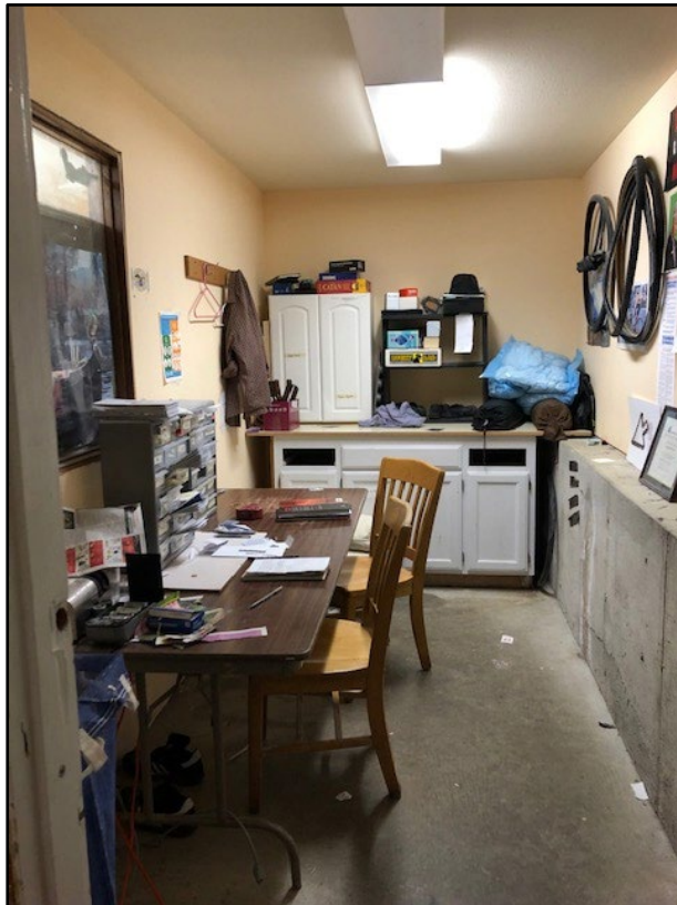
Figure 24. Basement room redeveloped as a break room. New concrete slabs are visible. Photo by author
