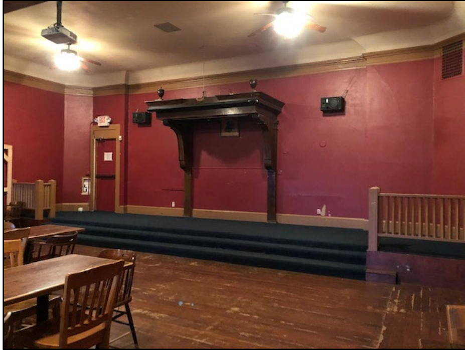
Figure 21. Dais and wooden canopy and railing retained on the second floor. Original floors exposed. A painted dog plaque just visible under the canopy originally held a Masonic plaque, and a “G” emblem on the canopy has removed at some point. Photo by author.
