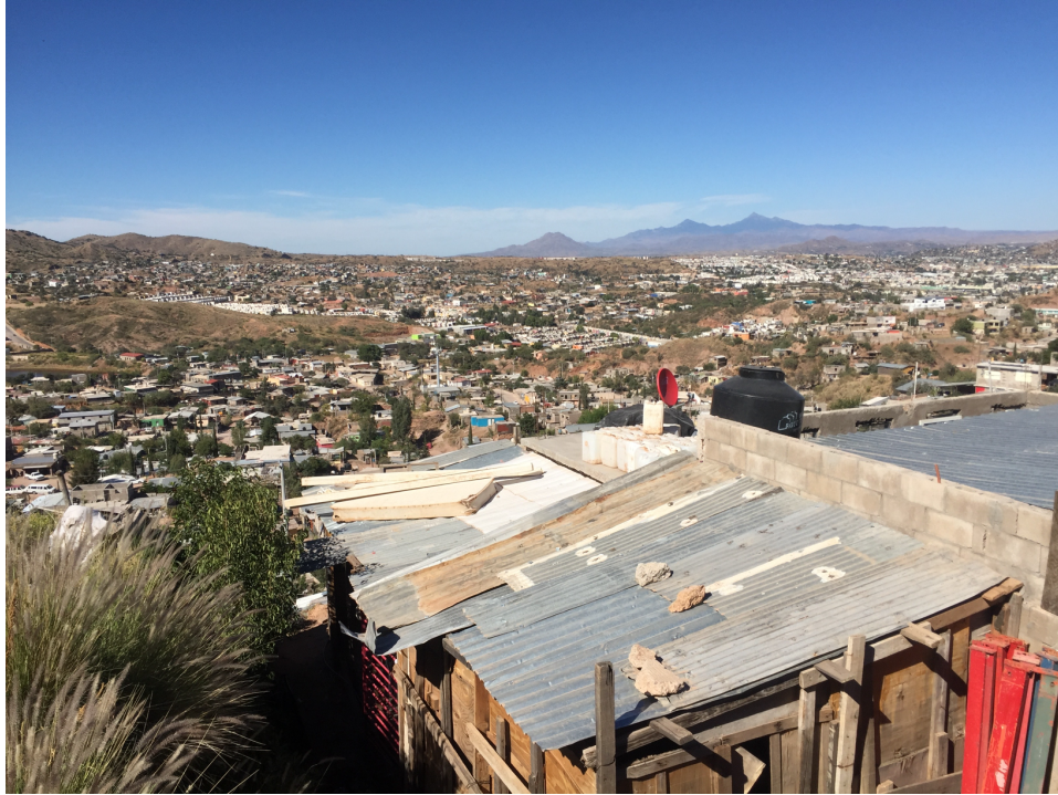
Figure 8. View to the north, overlooking a working-class neighborhood on the southwest outskirts of Nogales.
