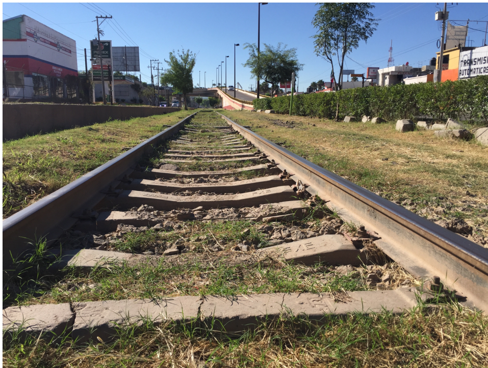
Figure 15. Southbound view of railroad tracks that bisect Nogales.
