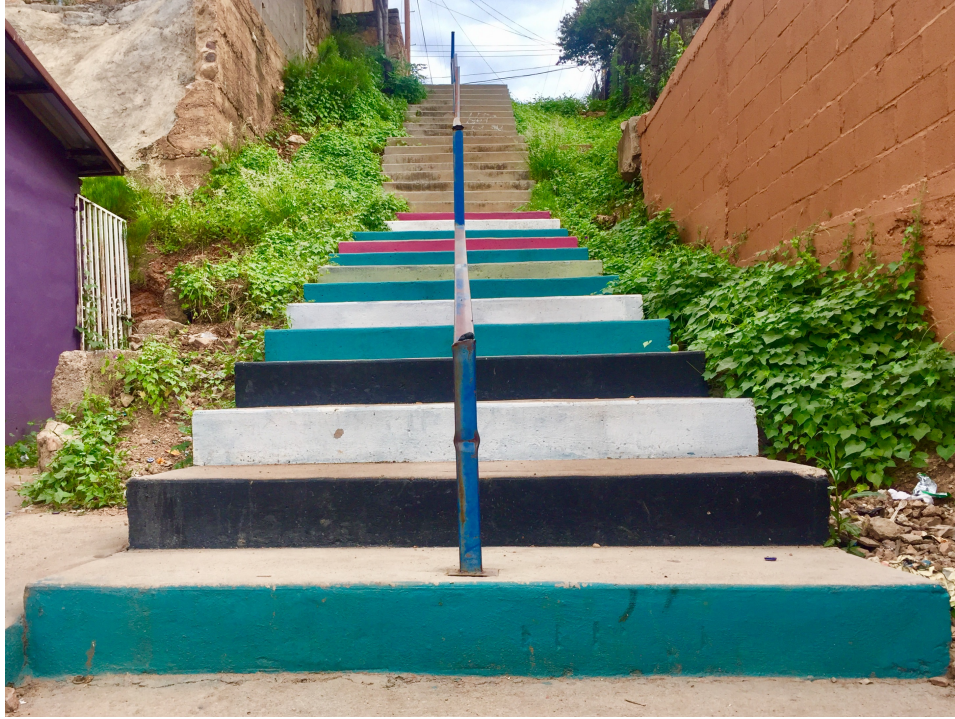
Figure 16. One of hundreds of escalinatas (outdoor stairs) in Nogales.
