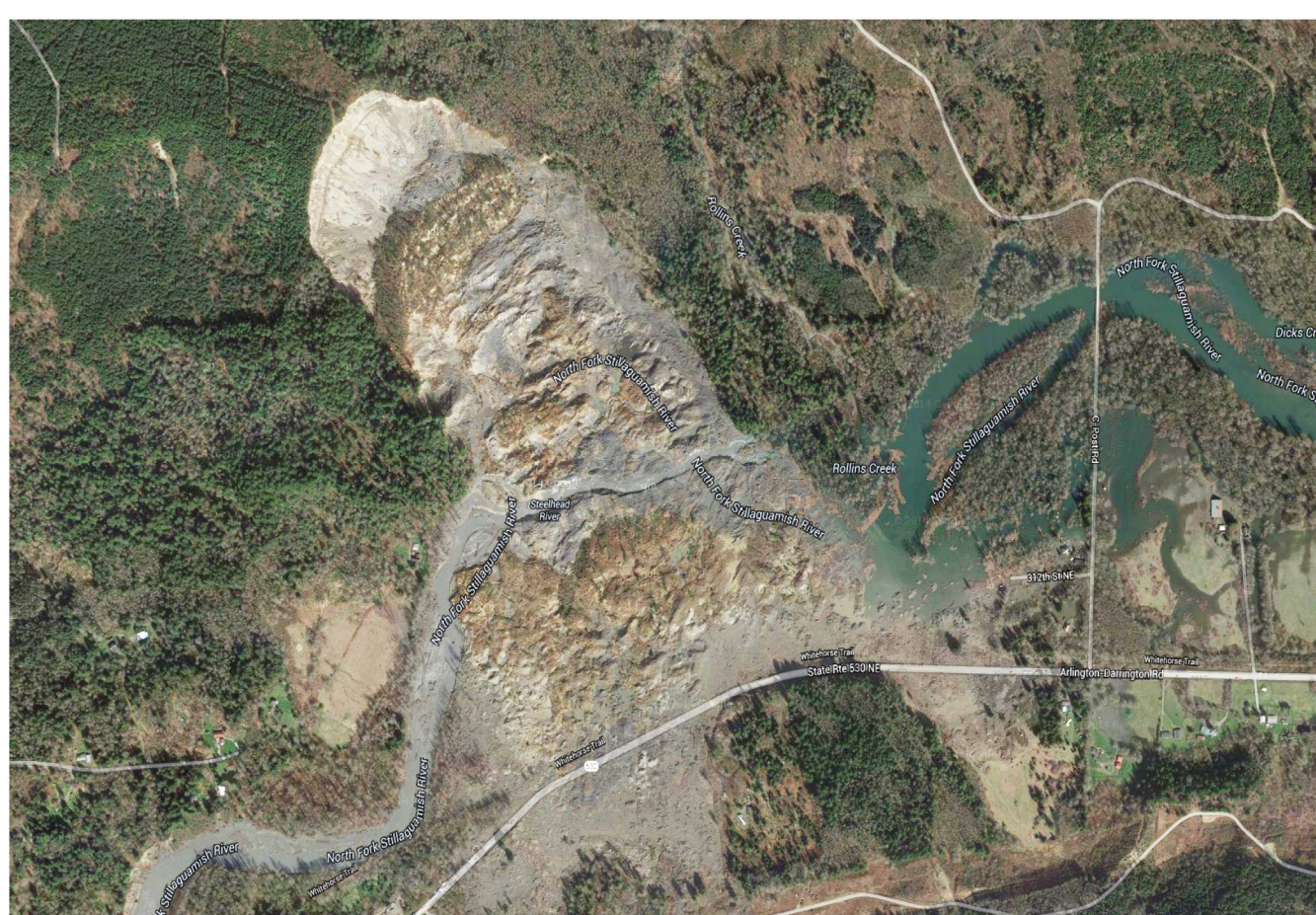
An aerial photograph of the Oso, Washington landslide showing the path of the slide and the Stillaguamish River.
