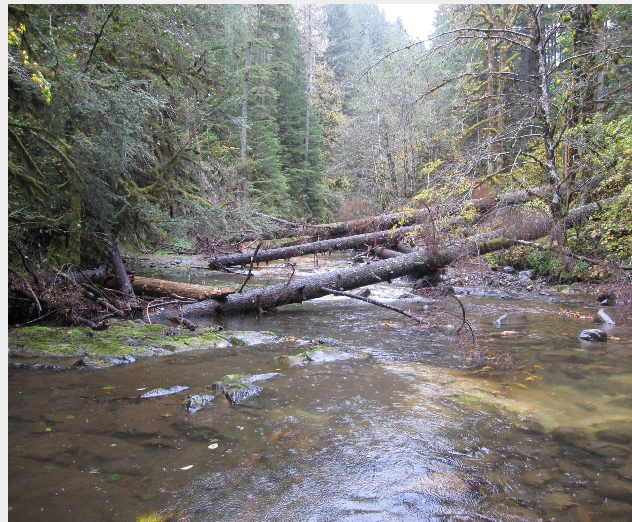
This is a whole tree structure tipped into the stream to recruit gravel, silt, and sediment, as well as to add to the complexity of the stream.
