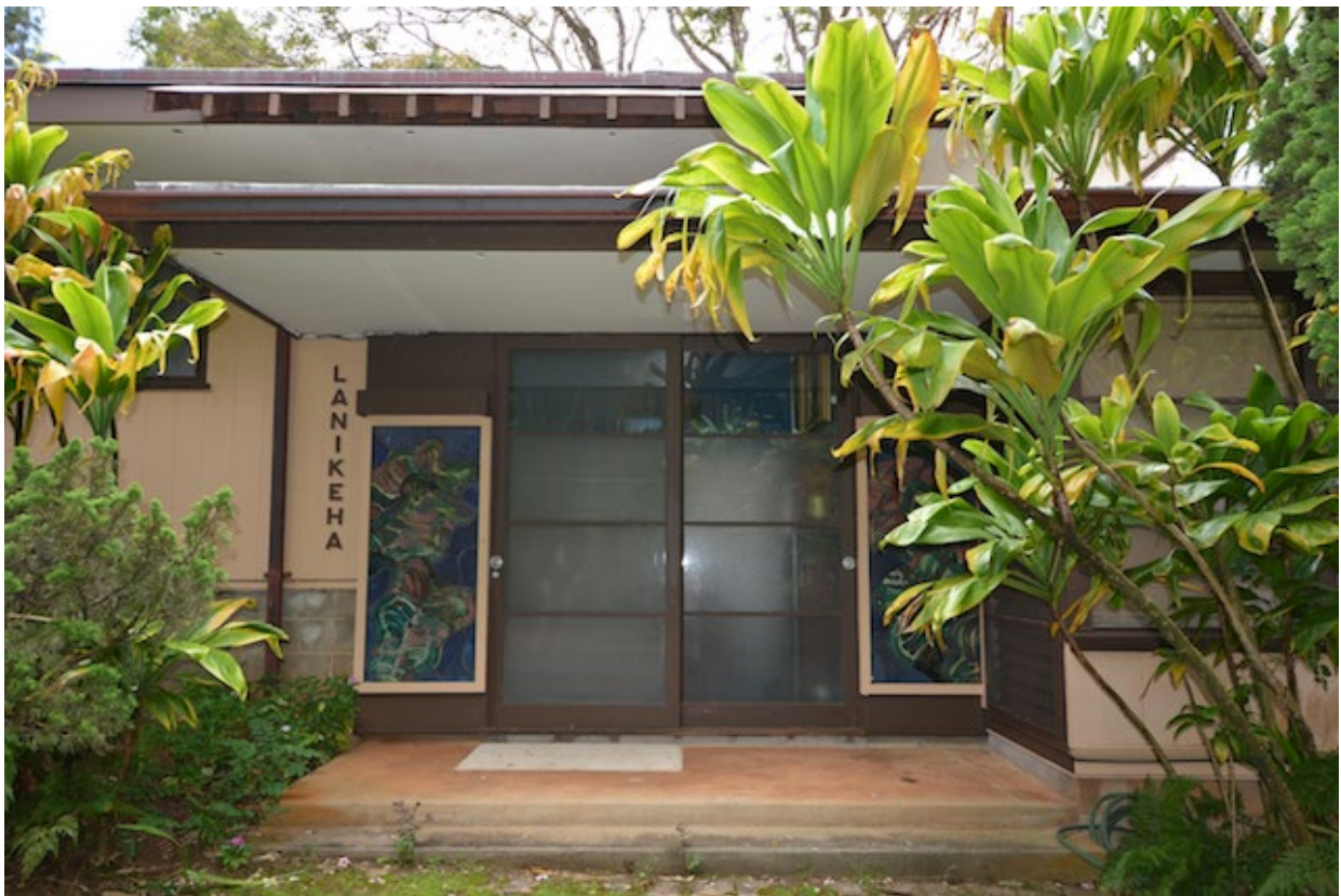
Figure 4.9 Sanford front entry with shoji doors of glass and redwood, 2013. Photo by the author.
