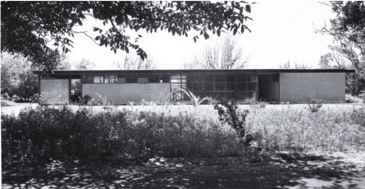
Figure 4.11 Milton Katz residence in Studio City, California, 1949. Architect: Raphael Soriano. Photo by Julius Schumann. Courtesy of the Getty Research Institute.
