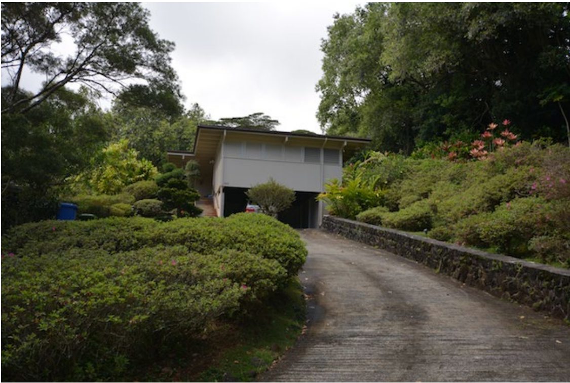
Figure 3.11 3610 Woodlawn Terrace Place, 2013. Photo by the author.
