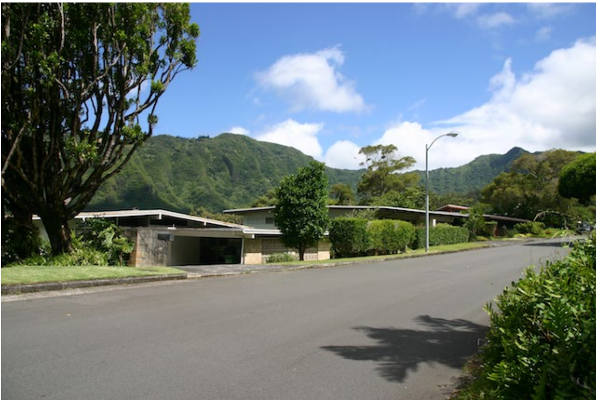
Figure 3.20 Street side view of 3637, 3635, and 3633 Woodlawn Terrace Place, 2013 facing northwest. Photo by the author.
