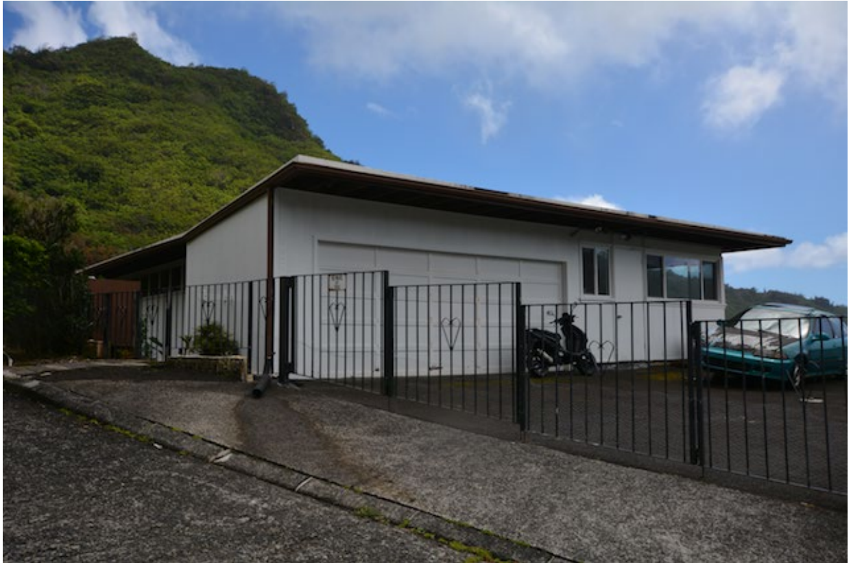
Figure 3.18 Vinyl windows at 3625 Anela Place, 2013. Photo by the author.
