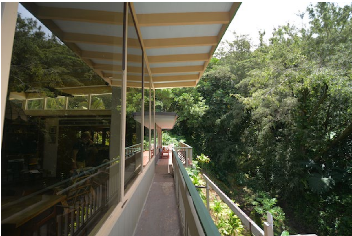
Figure 3.15 Living room window facing southeast, 3623 Manamana Place, 2013. Photo by the author.
