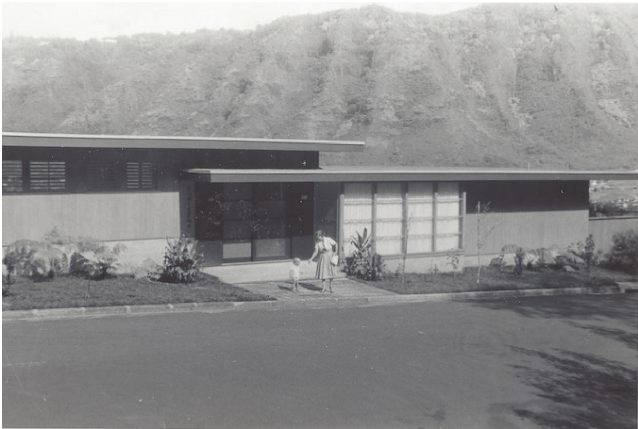
Figure 4.7 Sanford residence, front elevation, 1960. Photo by Wallace Sanford. Courtesy of Claire Sanford.
