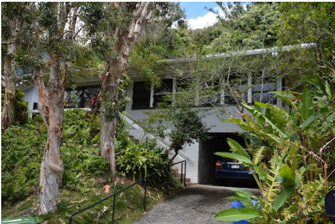
Figure 3.12 3618 Woodlawn Terrace Place, 2013. Photo by the author.
