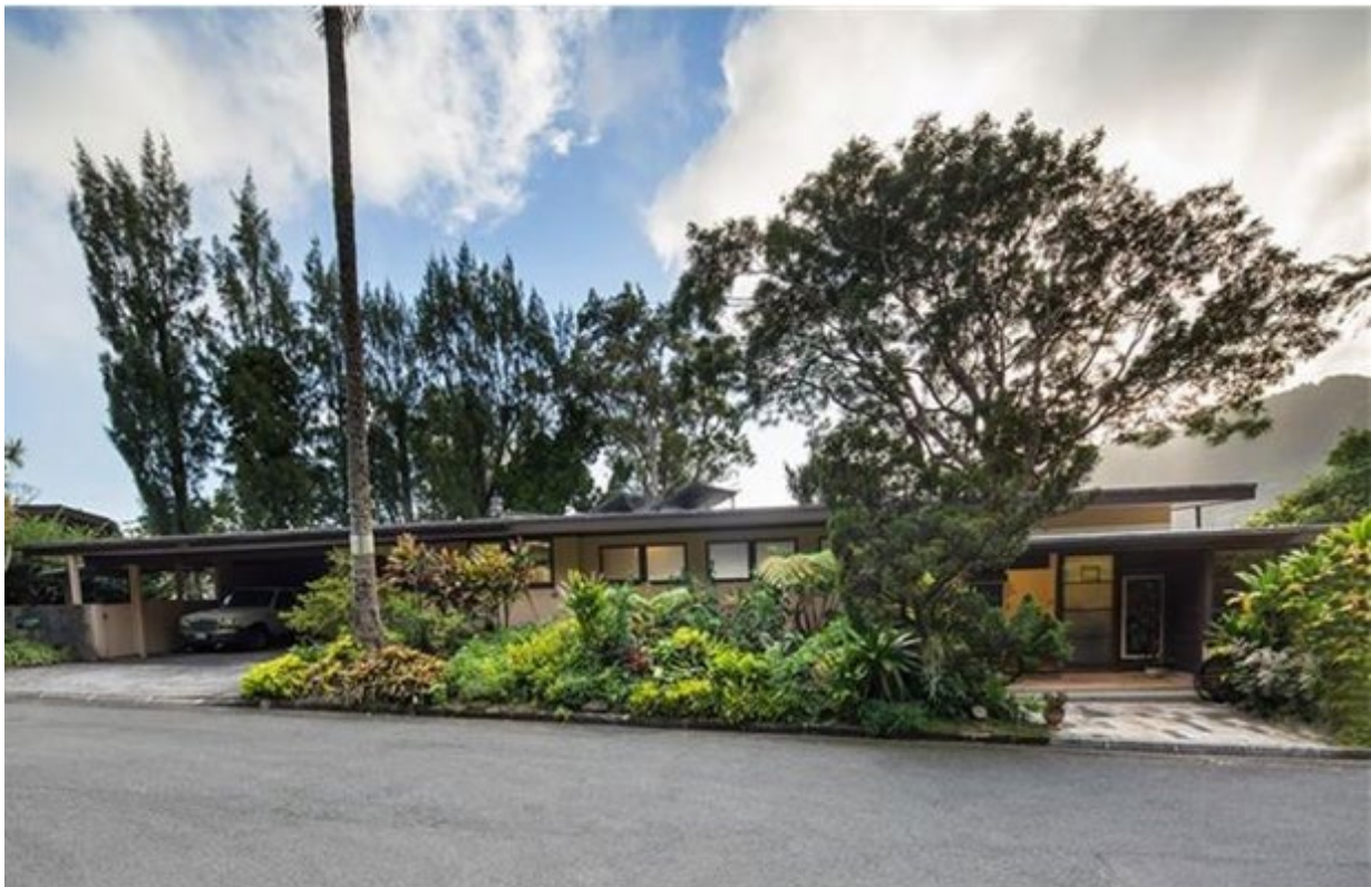
Figure 4.8 Sanford residence, front elevation, 2017. Courtesy of Sotheby's International Realty.
