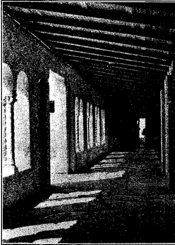
One of the "ambulatories" surrounding the interior court at the new arts building. This building was erected on the site of the burned women's gymnasium and is connected with the architecture building in the manner above shown. The colonettes supporting the arches were designed by students.
