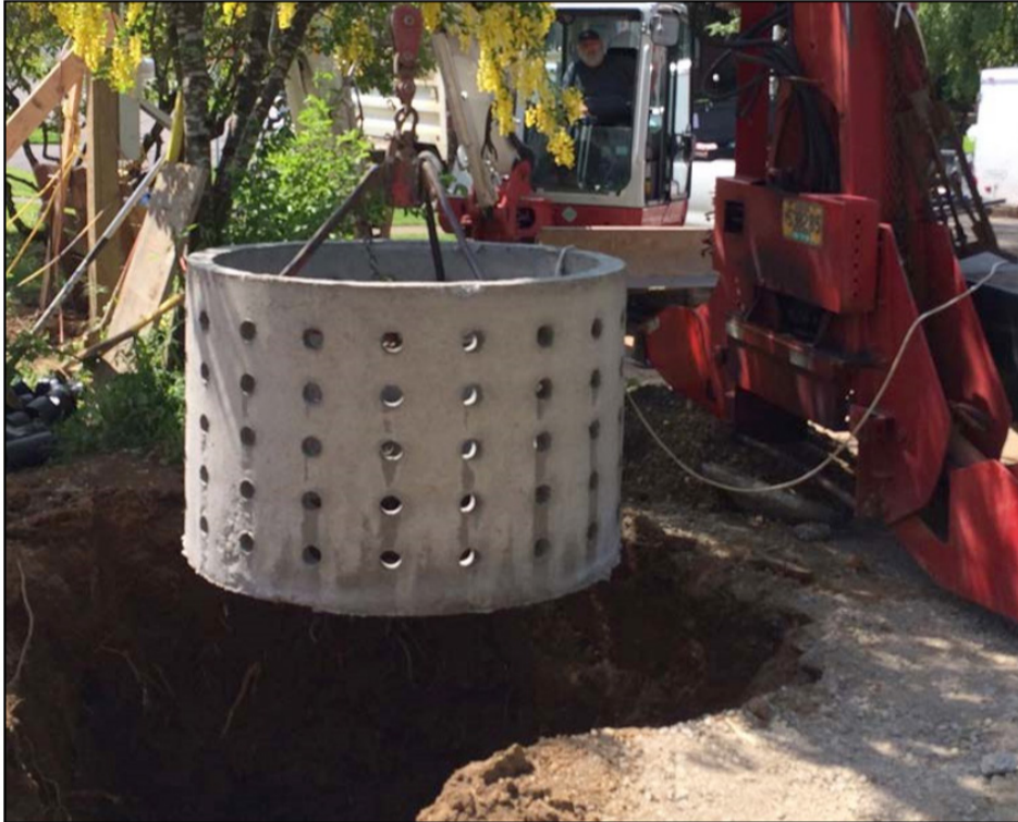
Figure 9: Drywell (SWMM Manual)
