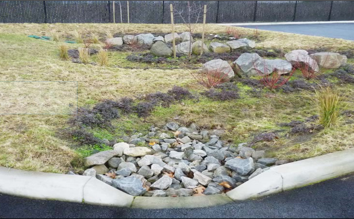
Figure 4: Swales (SWMM Manual)
