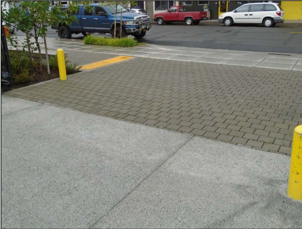
Figure 8: Pervious Pavement (SWMM Manual)
