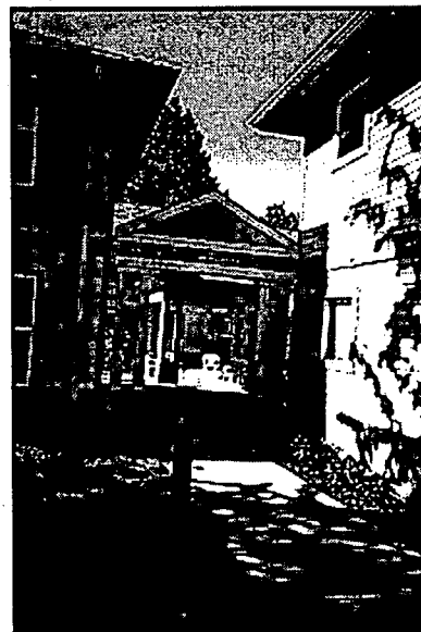
D. Emphasizing the front entrance of a multi-dwelling complex with an architectural element such as a portico, trellis, or arch.
