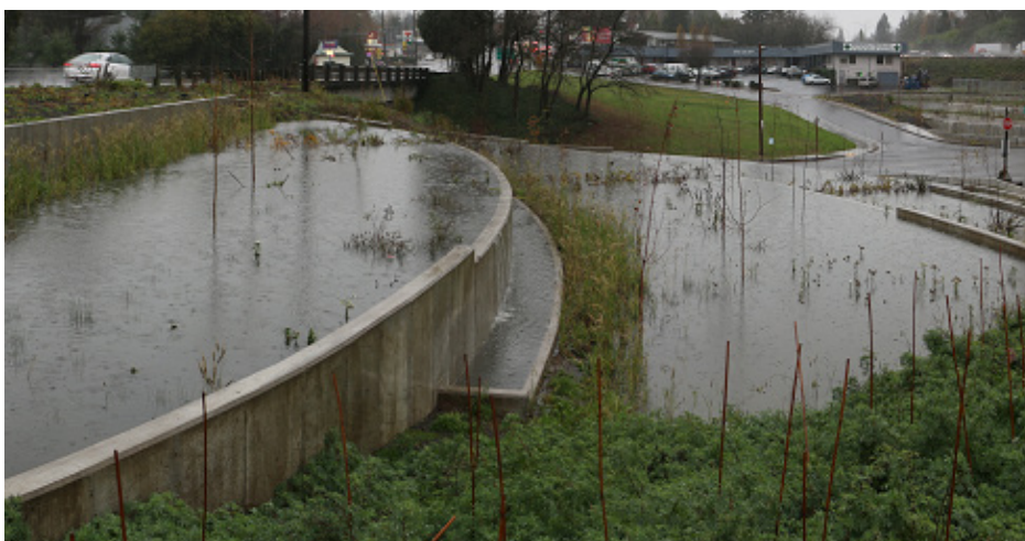
Figure 28: Rain gardens can slow water runoff as well as absorb pollutants. Source: Portland BES
