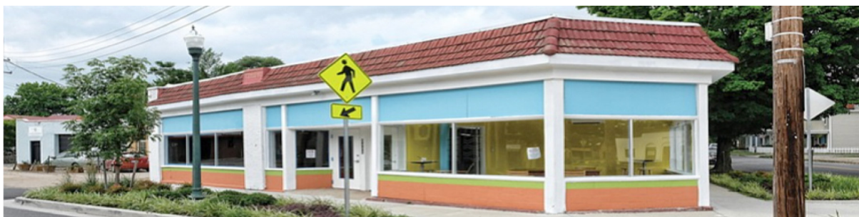
Figure 8: Before and after activation of the storefront space
