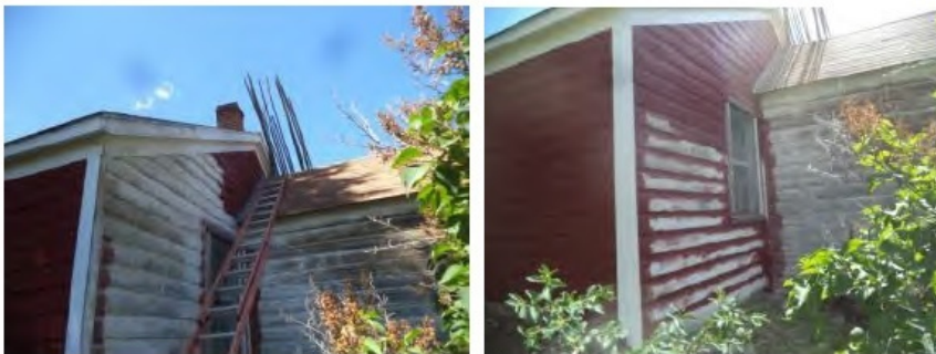
The northeast side is scraped, primed, and painted.
