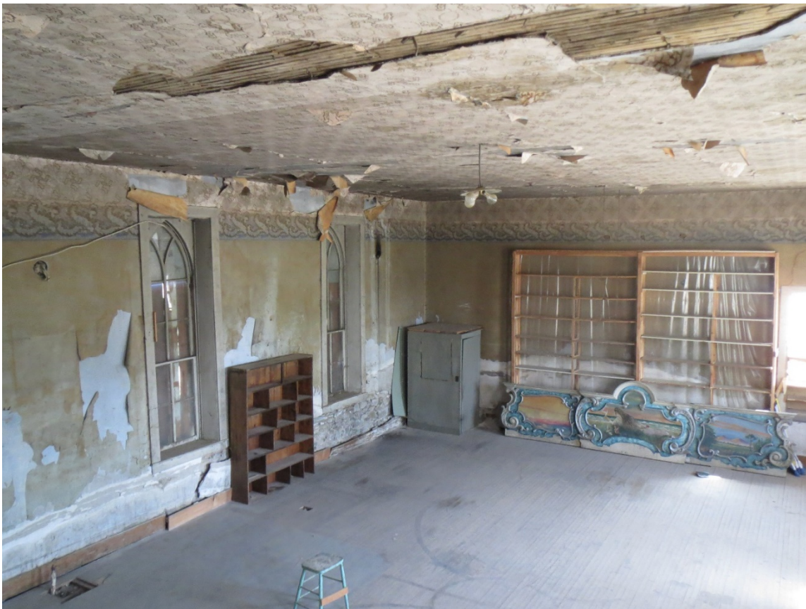
Figure 2.17. Methodist Church interior. Note the painted gymnasium floor and intricate wallpaper of lath plaster ceiling, August 25, 2016. (Photographed by K. Geraghty)
