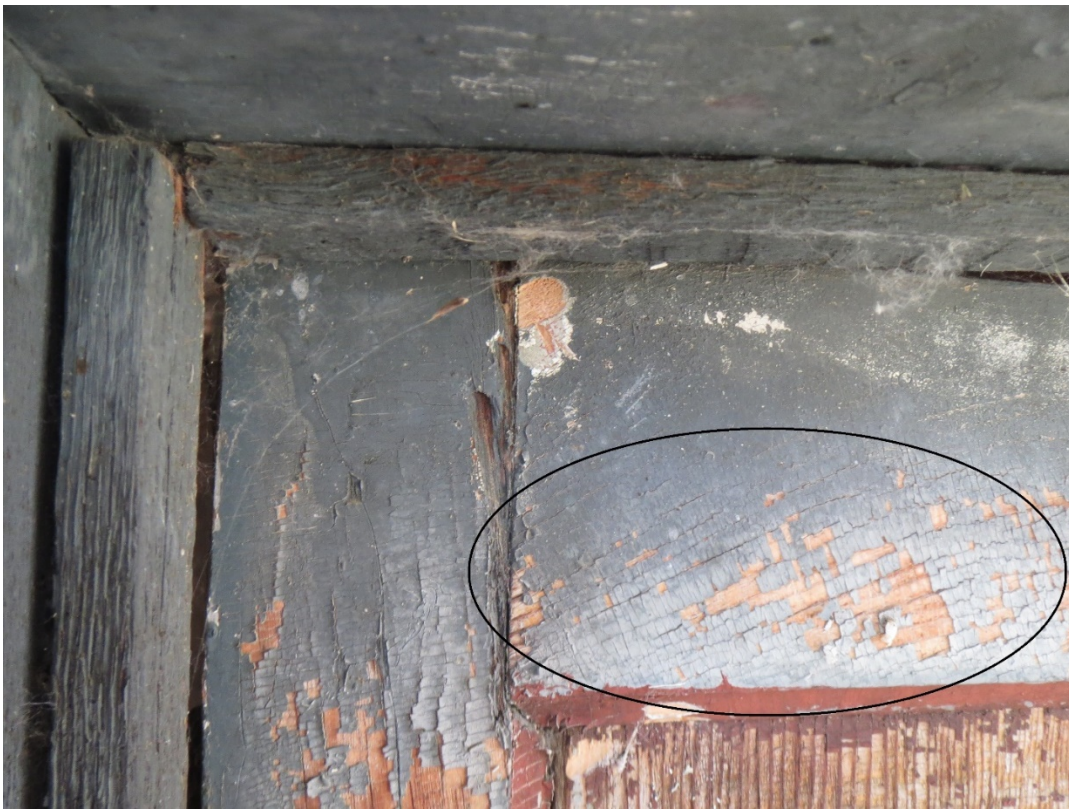
Figure 6.2. Example of "alligatoring" at Green Fronts. Photo by K. Geraghty August 24, 2016
