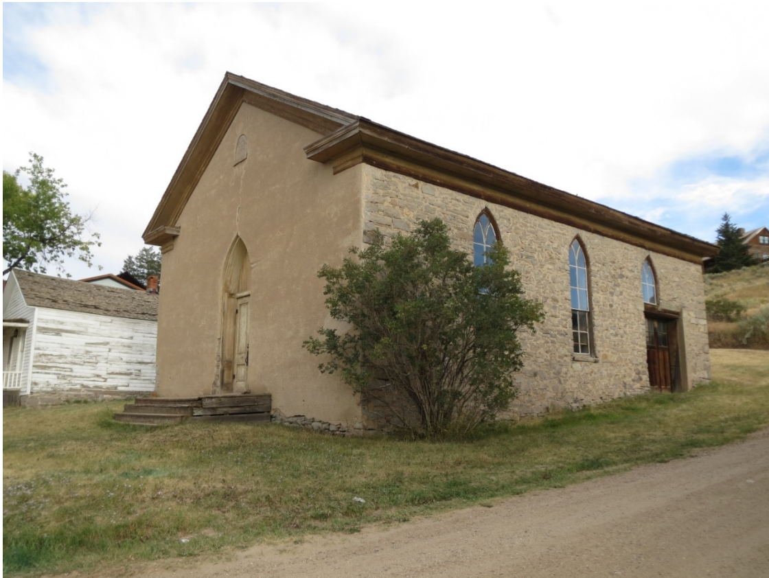
Figure 2.16. Methodist Church with Daems-Corbett House in background, August 25, 2016 (Photographed by K. Geraghty)
