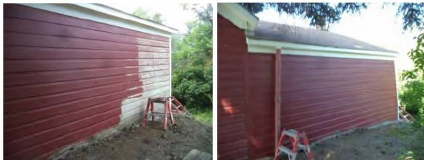
The east side is scraped, primed, and painted.
