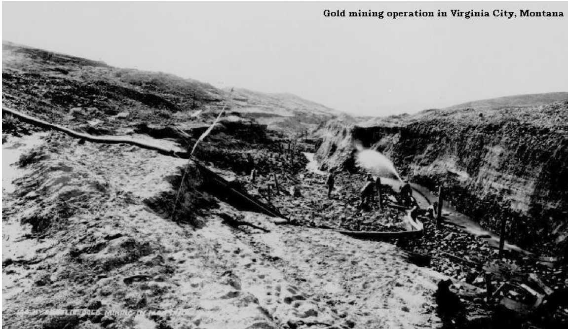
Figure 2.5. Hydraulic mining operation in Virginia City, Montana (Photographer William Henry Jackson, 1867, Library of Congress #2005686471)
