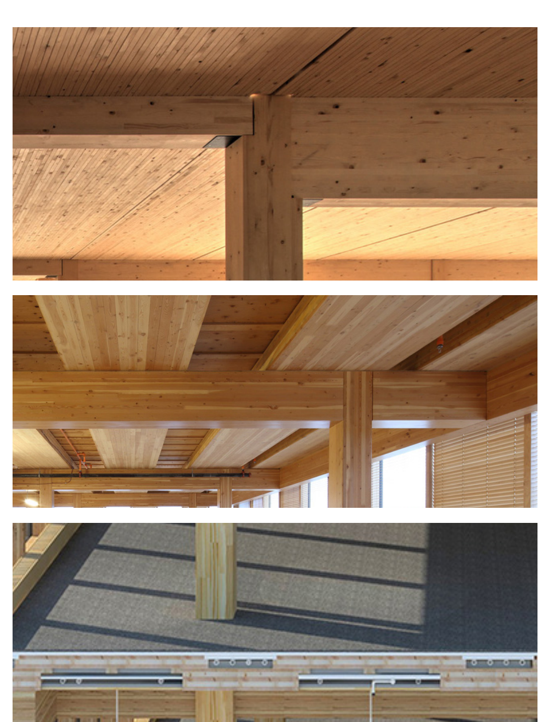
Gravity Performance Continuous CLT Deck Concrete Topping Layer Glulam Beams
