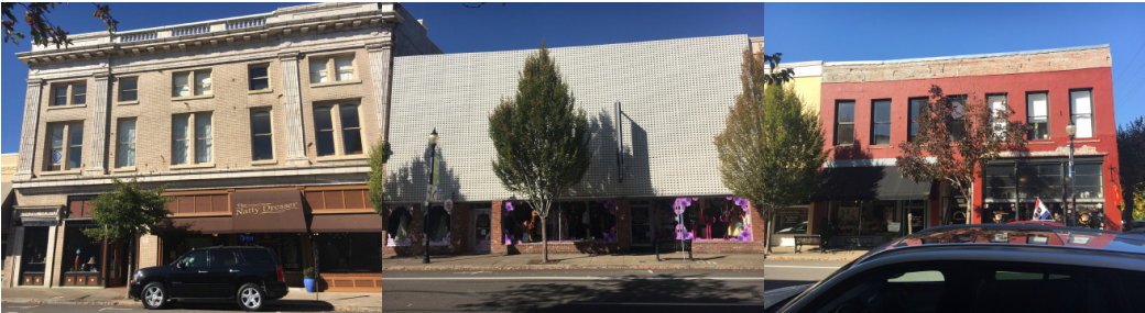
Views looking North across 1st Street
