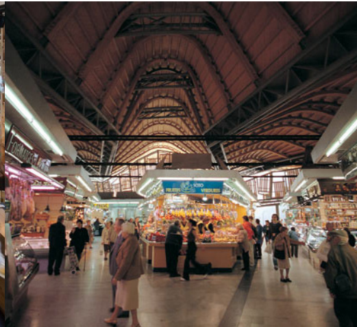
Roof vaulted space
