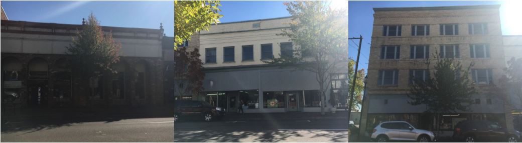
Views looking South across 1st street
