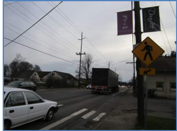
Crosswalk at 10 th Street is signed but not signaled
