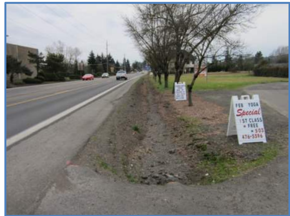
99W south of 12 th Street: part of the City's incomplete sidewalk network
