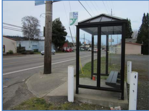
Shelter for northbound travelers at 9 th Street on Highway 99W
