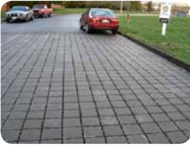
An example of permeable pavers
