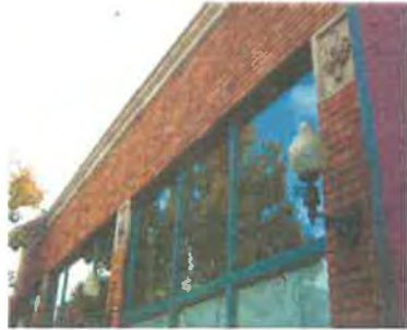
Building lighting, medallions, and transom windows
