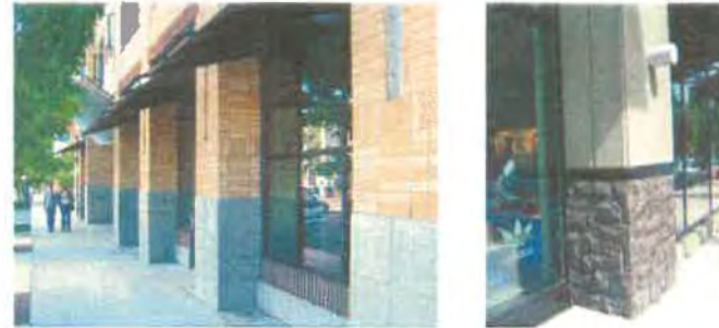
Pilasters can help break up a building facade, while defined footings can help anchor a ground floor at a human scale.
