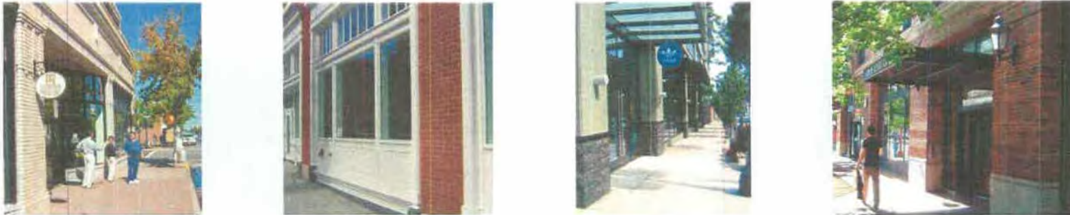
Distinct architectural bays can help break up a building while distinguishing its ground floor and improving its appeal to passersby.
