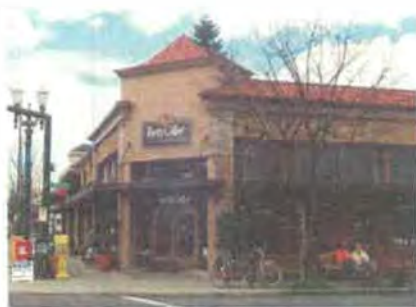
Chamfered buildings and elements such as turrets or cupolas can help define corners and intersections as important gathering places.
