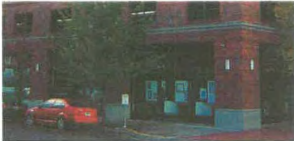
Belt course, here distinguishing ground floor and second floor
