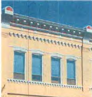
Windows with unified lintels and sills
