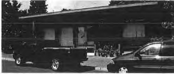
Also represented is an interesting modern one-off of a style not found elsewhere in Downtown. This post-and-beam commercial building appears highly-organized and logical. It features prominent storefront windows and a flat roof form with deep overhangs.
