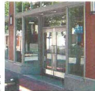
Prominent, recessed entry that features transom windows, large glass entry doors (with kick plate), and flanking windows.
