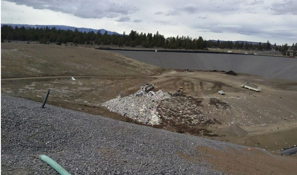
Figure 7: Truck unloading garbage from Redmond at the Deschutes County Knott Landfill.
