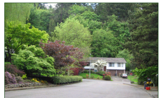
Split-level ranch home on sloped lot is dominated by mature trees.
