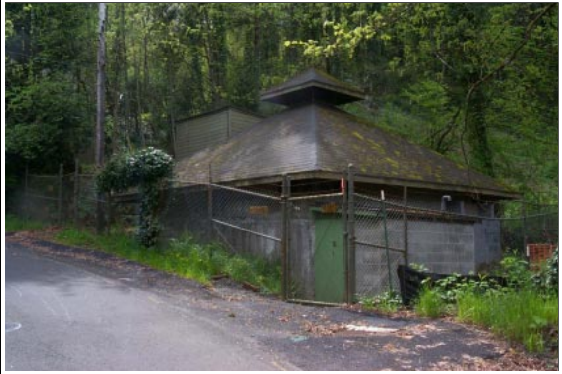
Glenmorrie Water Cooperative Pump House and Water Storage Facility
