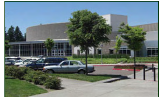
The entrance to Lakeridge High School presents a modern façade of concrete and glass.
