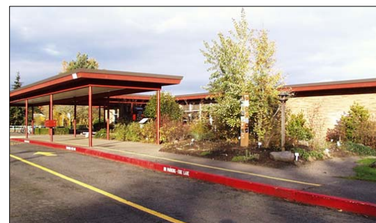
Palisades Elementary School opened in 1958 and exhibits the influence of the "modern" /international style with its low profile, flat roofs and overhanging eaves, lack of ornamentation, and a functional approach to design..
