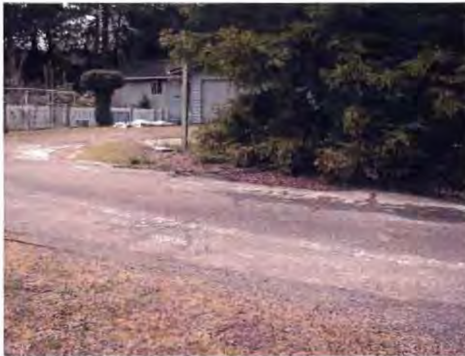
PCI Range 0 – 29 Hemlock Street – PCI 27 (Has been rehabilitated in 1 st year program) Current PCI - 97
