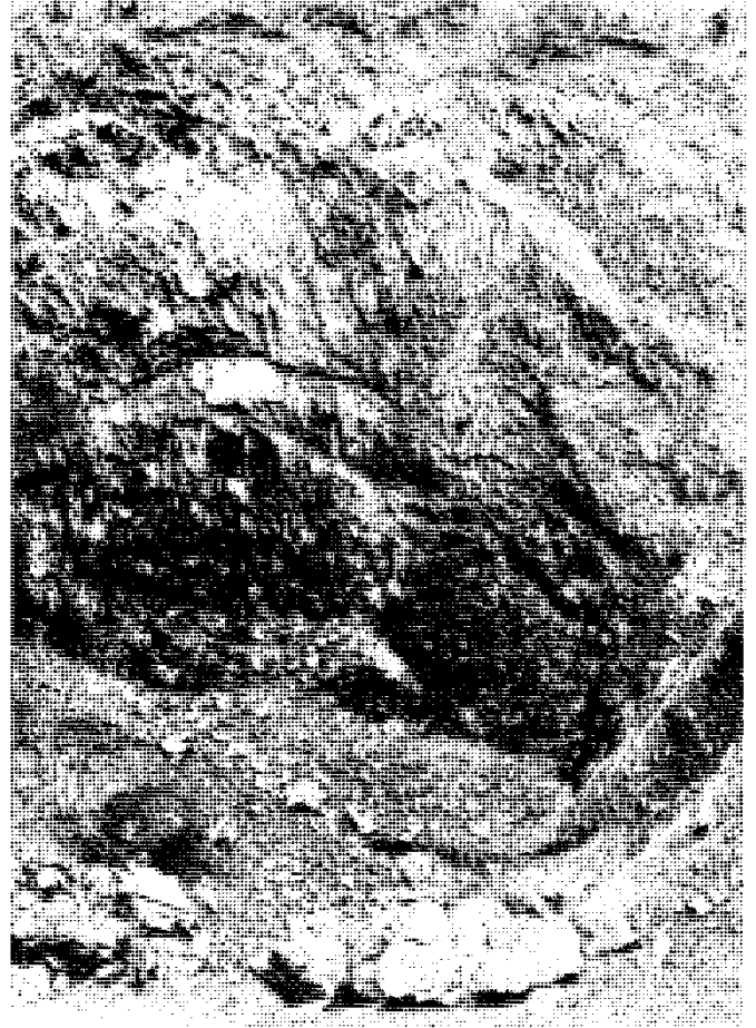
Figure 5b. Site 123. Note man in foreground for scale. Hazards include highwall heights, large loose boulders on sloping fracture planes, and loose overburden at top of quarry.
