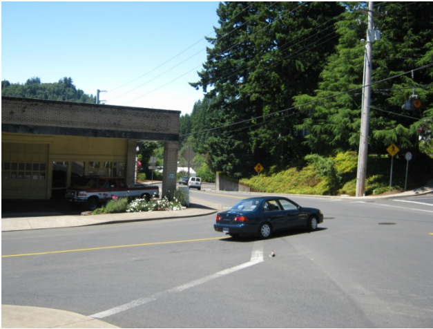
Vehicle turning left onto Business Loop 20 from Main Street. Building pillar restricts sight distance.
