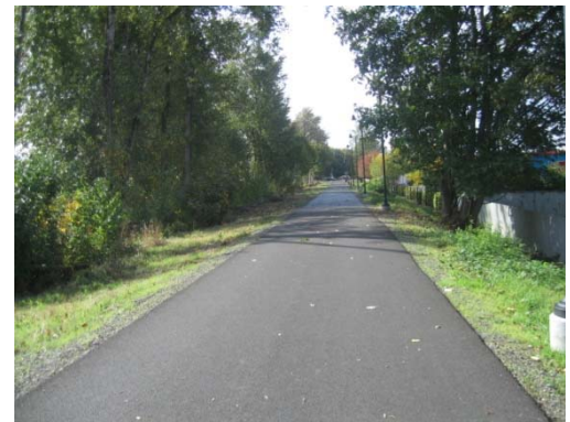
Example of a paved multi-use path
