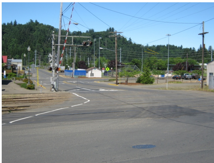
Rail Crossing at Butler Bridge Road and 1 st Street
