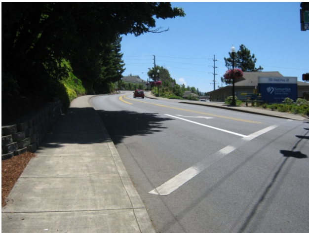
Sidewalks on Business Loop 20 near A Street
