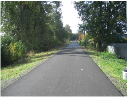
Example of a paved multi-use path
