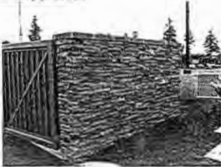
Figure 8: Masonry screening that is architecturally consistent with the principle building hides garbage collection and mechanical equipment areas.
