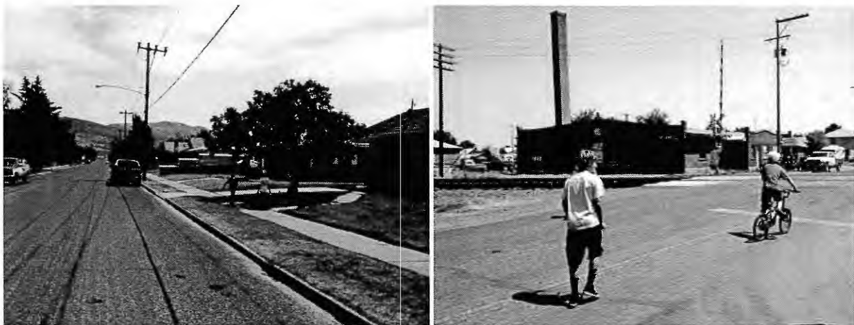
Exhibit 3 Examples where sidewalks are present along Myrtle Street (left) and absent along 9 th Street (right)
