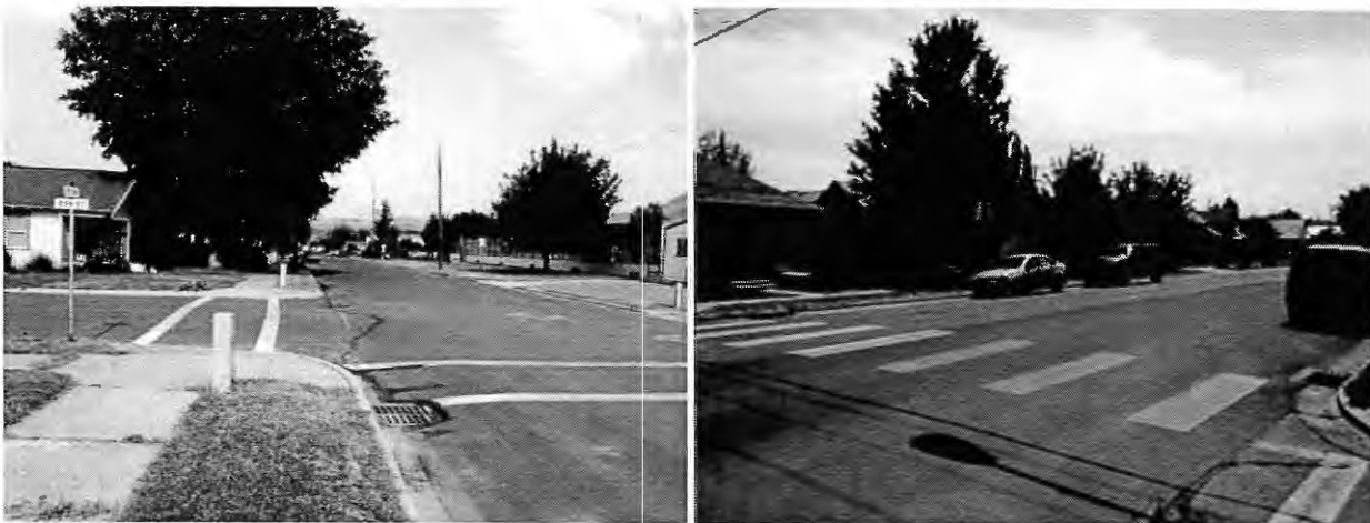
Exhibit 5 Examples of transverse crosswalks near Brooklyn Elementary School (left) and continental crosswalks on US 30 (Elm Street) at Myrtle Street (right)
