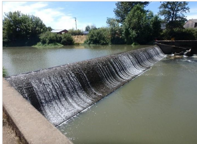
Figure 4: The 2.9 m tall drop structure in Monroe acts as the furthest downstream fish passage barrier on the Long Tom River. Image taken by author in 2015.
