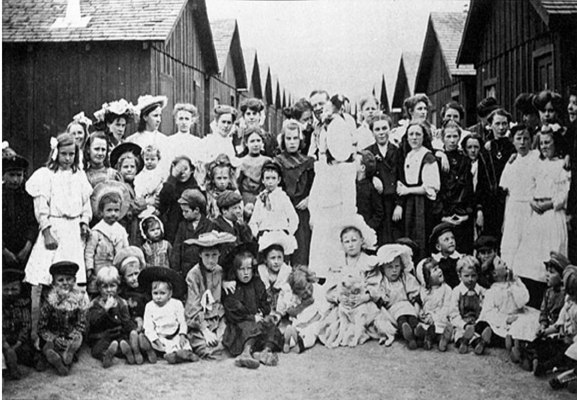
Figure 10: Close quarters in Hamilton Square. (Image: OpenSF History.)
