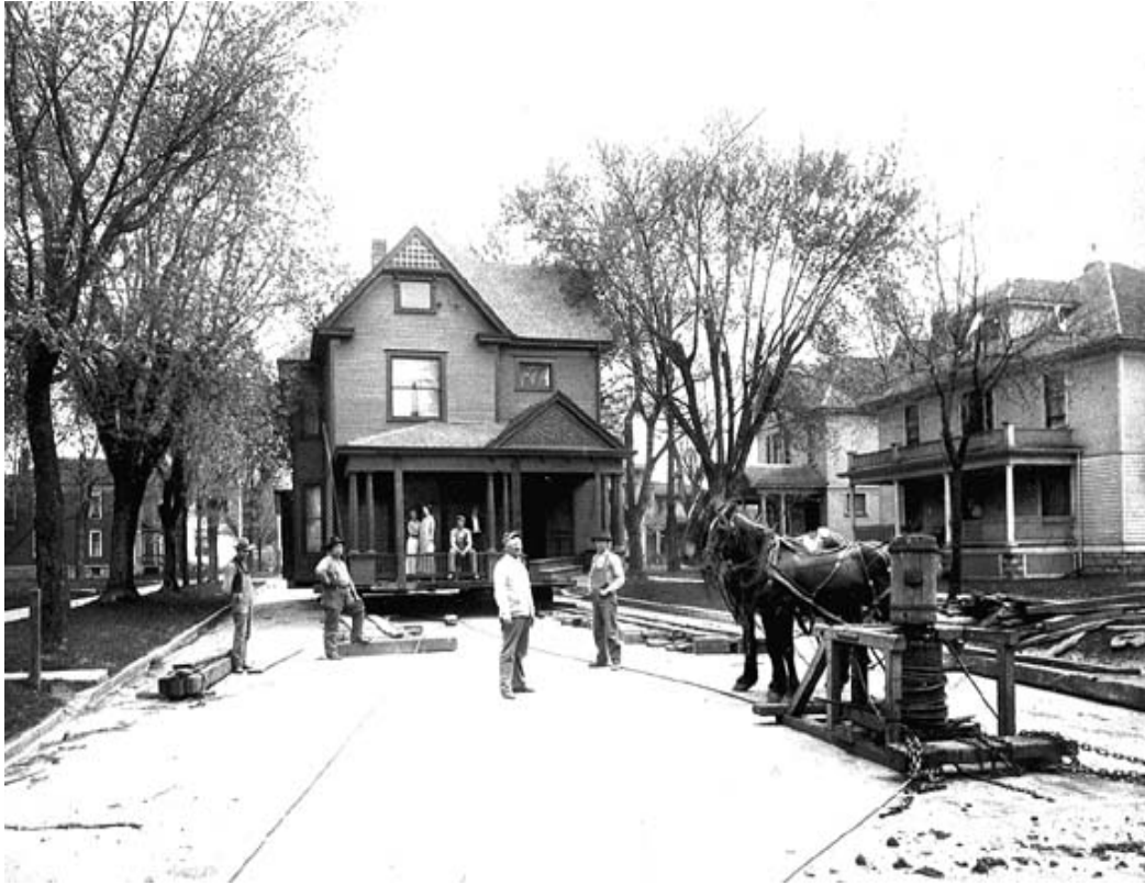
Figure 16: House moving in Michigan with a horse and capstan. (Image: Diane Donovan).
