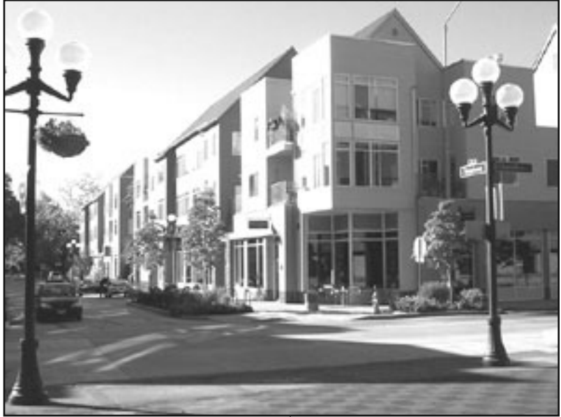
Broadway Place in Eugene, built in 1999, includes transom windows above building entries and large, regularly spaced windows
