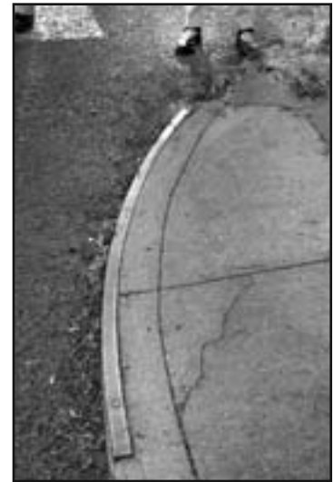
Many corners in downtown Junction City still have their historic buggy guards
