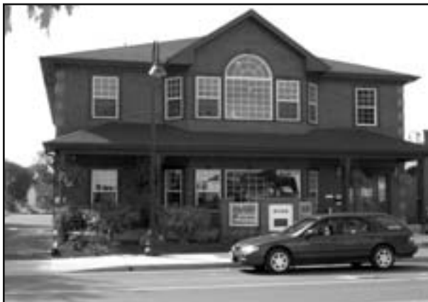
A small access drive (left of picture) takes drivers to parking located at the rear of the building. This allows the building to be close to the street
