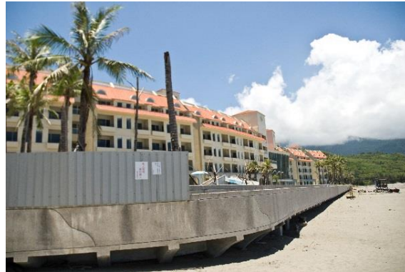
Figure 4: A photograph of Miramar Resort, with construction walls still up. (Personal photograph, 2014)
