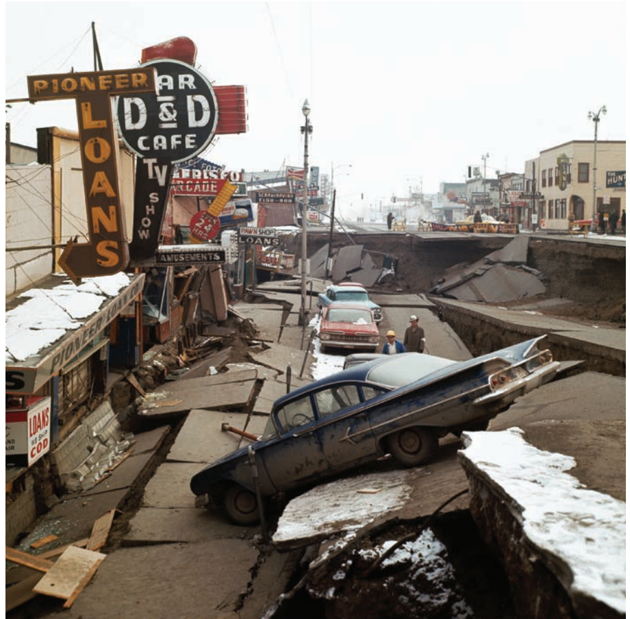
Alaskan Aftermath The March 27, 1964, Anchorage earthquake—which dropped this street some 20 feet below its normal level—was stronger than the 2004 Indian Ocean quake that caused a tsunami responsible for more than 200,000 deaths.
