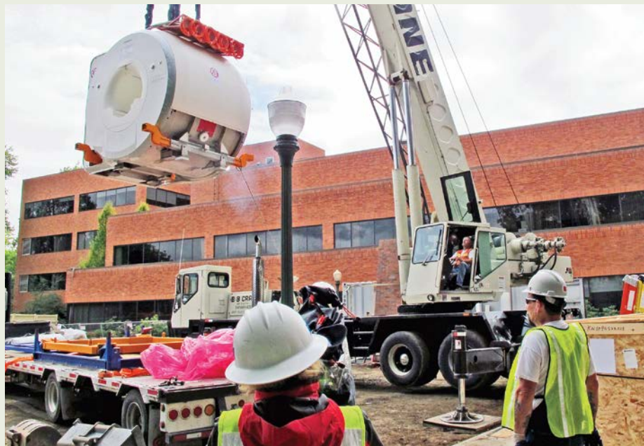
Six Tons Aloft A crane crew hoists a new research-grade magnetic resonance imaging (MRI) machine into the Lewis Integrative Science Building, which opened in October. Cognitive psychologists, physiologists, and researchers in other fields will use the $2.7 million scanner to create detailed images of the brain and body.
