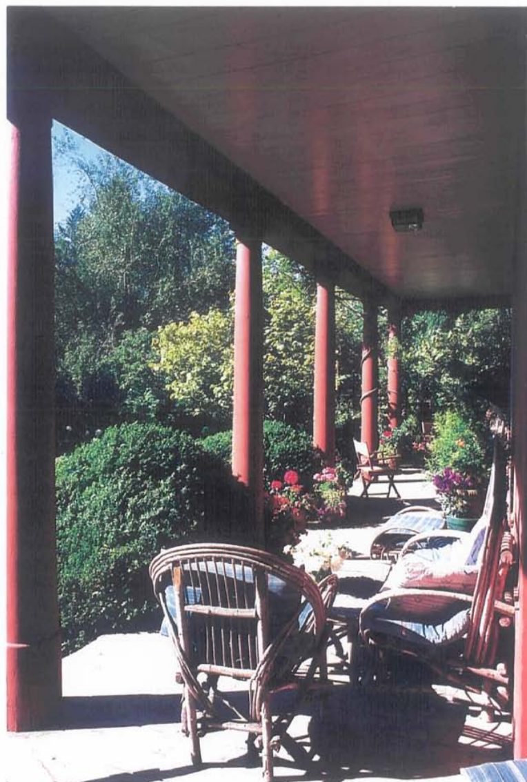
5.6 The south porch, looking southwest.
