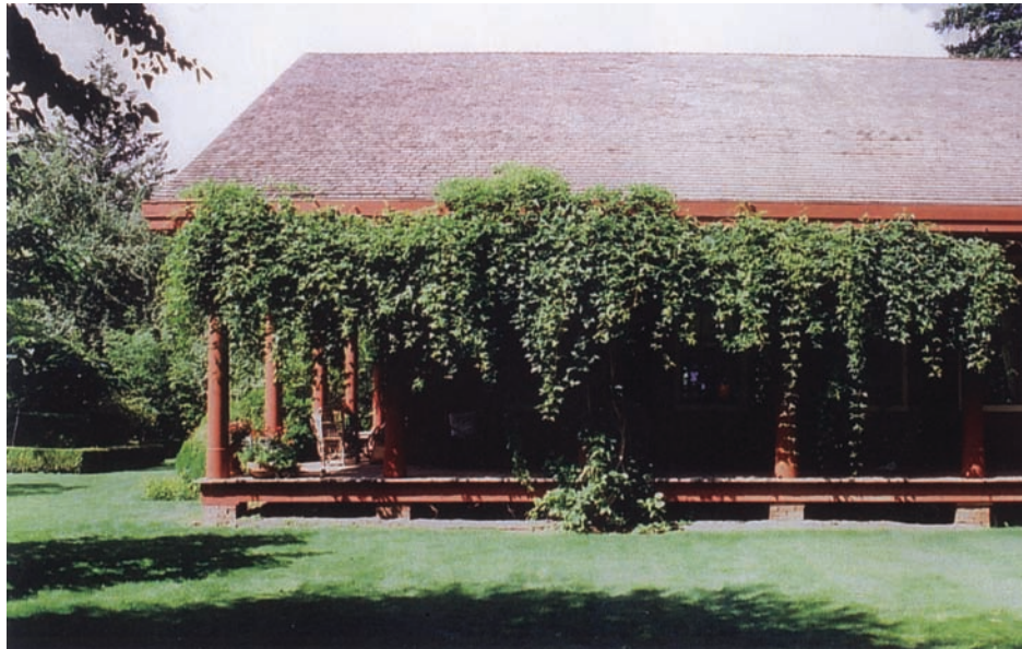
2.8 The southern half of the eastern façade.
