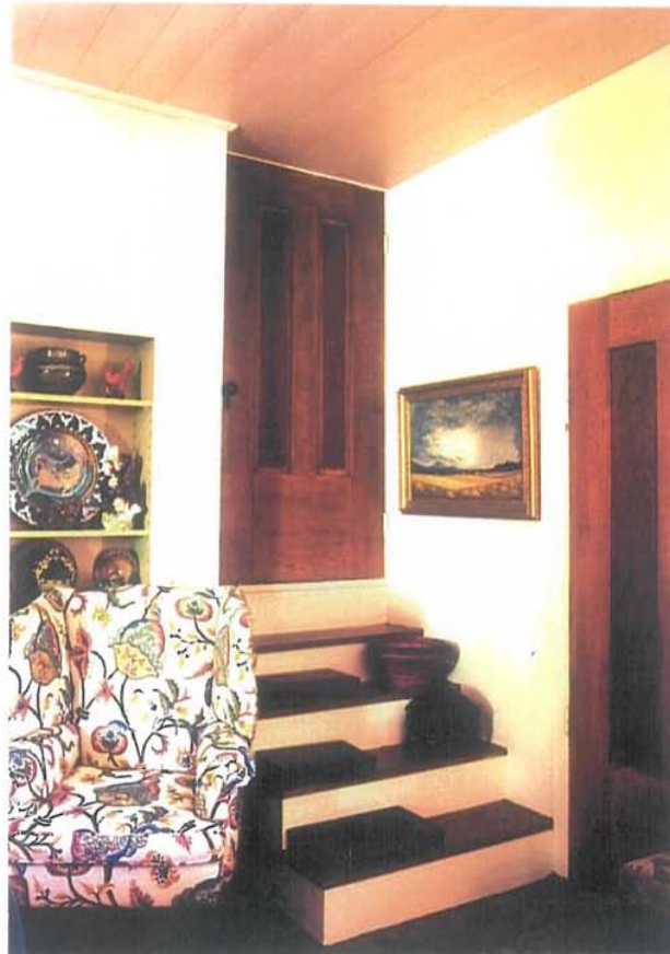
2.13 The northeast corner of the living room: coordination of attic door, stair, exterior door trim, and exterior door.
