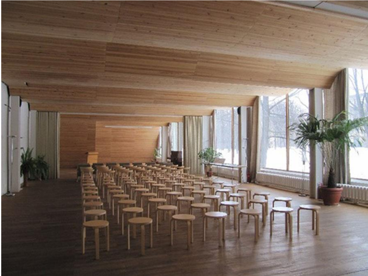
Viipuri Library, Lecture room with undulating acoustic ceiling
