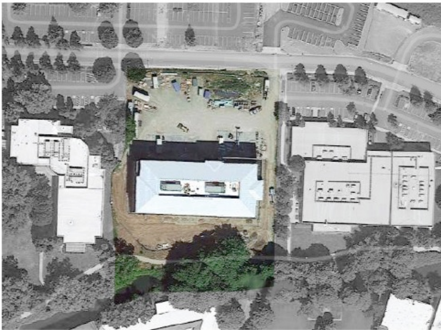
Figure 13: Aerial view of the research site while under construction, source: Google Maps, 2014.
