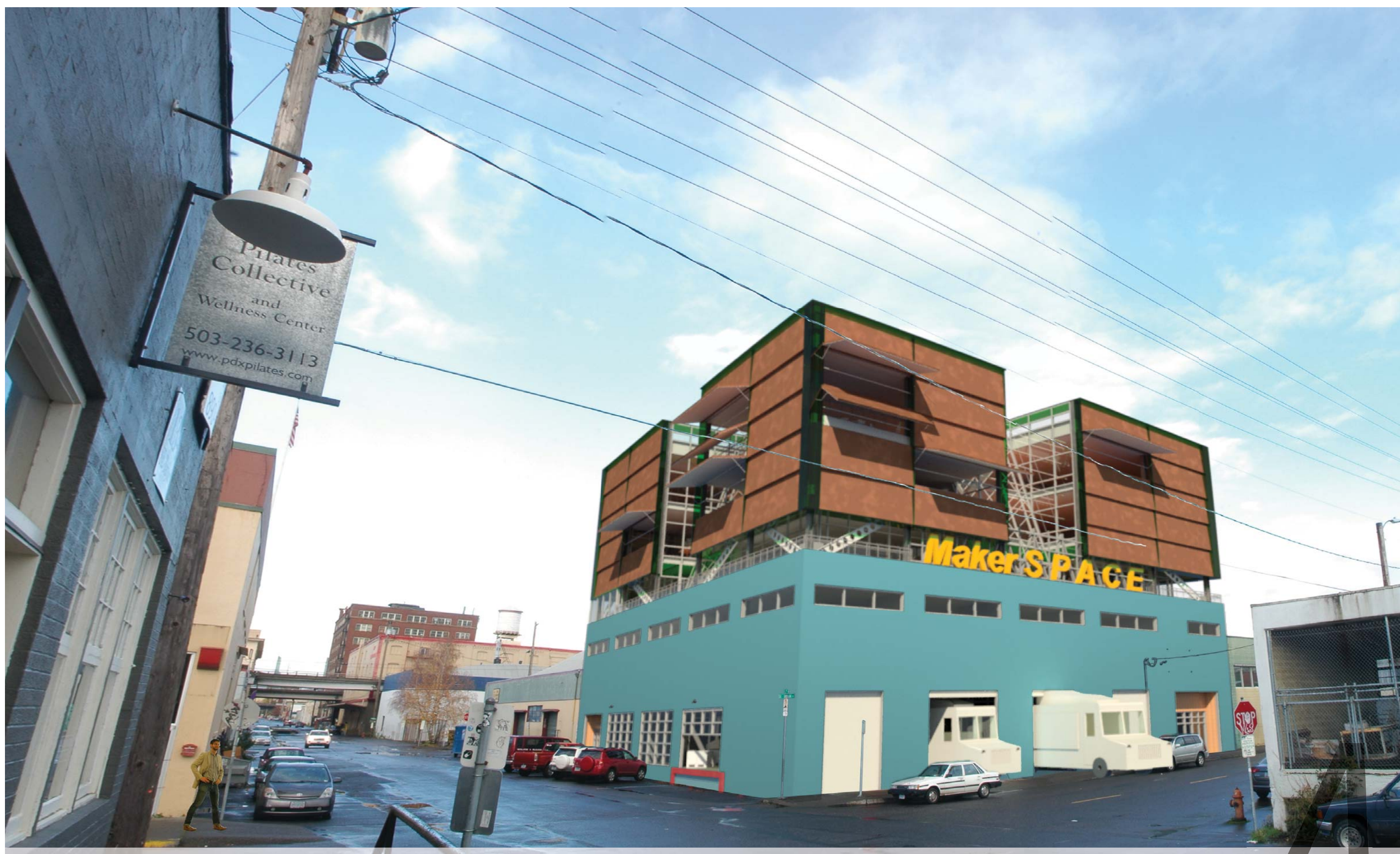
Exterior Perspective | Southeast Second Street - Adaptively re-used base, with new light frame structure above and fully user-operable metal panels for air.
