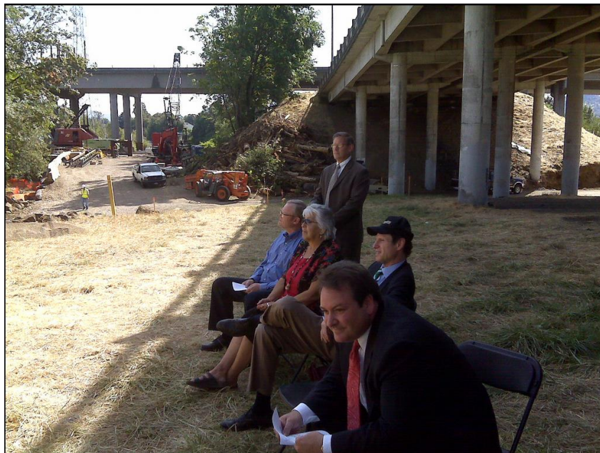
Officials wait for their turn at the podium during the Willamette River Bridge groundbreaking event.
