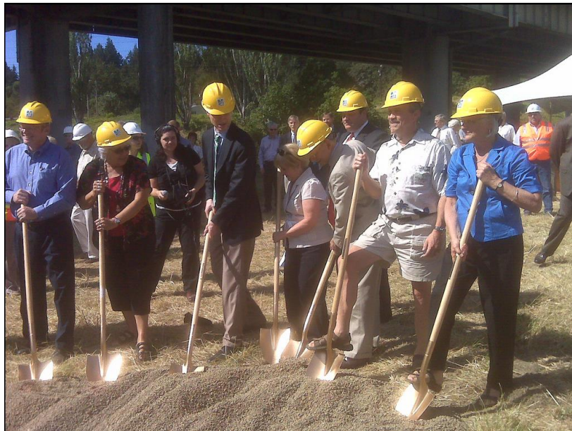
Officials break ground for the Willamette River Bridge project on Interstate 5 in Eugene.
