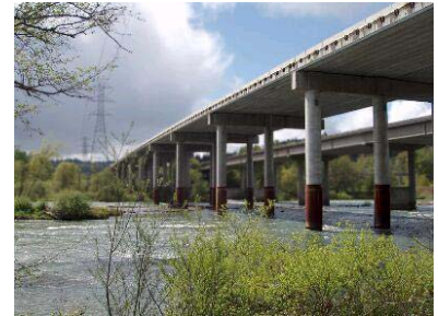
Existing bridge conditions
