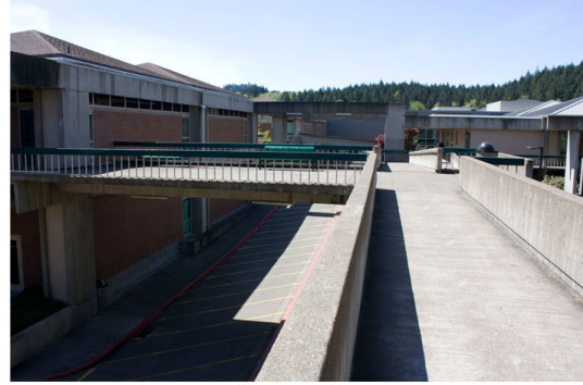
Connection (Lane Community College)
