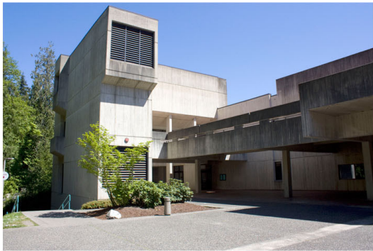
Exposed mechanical systems (Evergreen State College)
