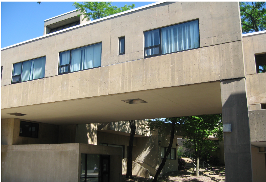
Figure 23 - Covered portion of one raised walkway type at SUNY Old Westbury
