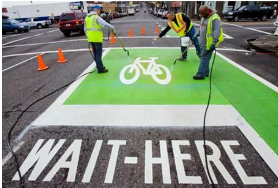
Figure B-14. A bike box is created in Portland, Oregon; photo from The Oregonian ; 21 Mar. 2008.
