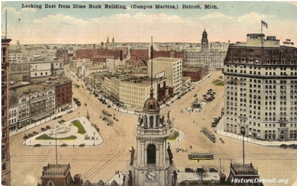
Figure 4.5. Old City Hall in foreground looking east across Cadillac Square to Wayne County Courthouse.
