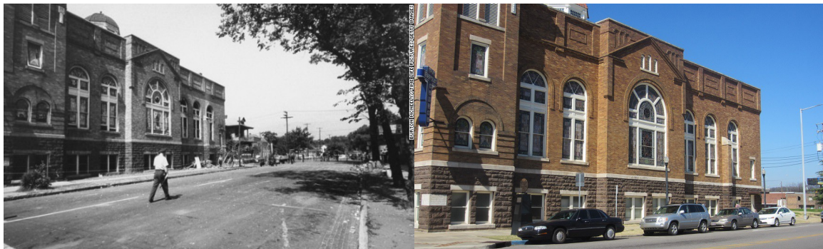
Looking northwest (September 15, 1963/ March 20, 2014)
