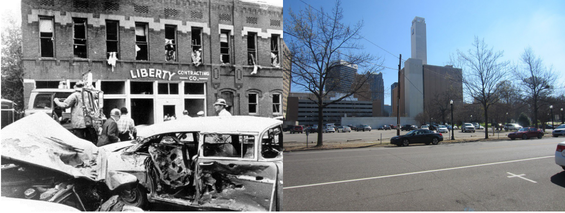
Looking East across 16 th Street (September 15,1963/ March 20, 2014)
