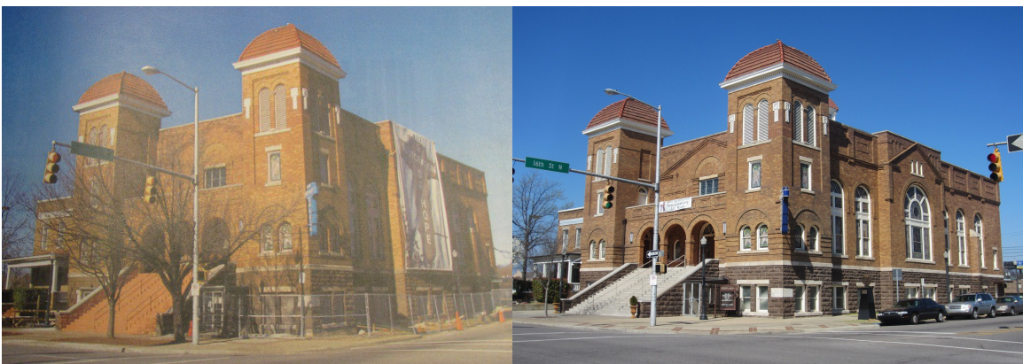
The church before and after the removal of the orange tile on the steps (2006, courtesy of Architecture Works/ March 20, 2014, courtesy of the author)
