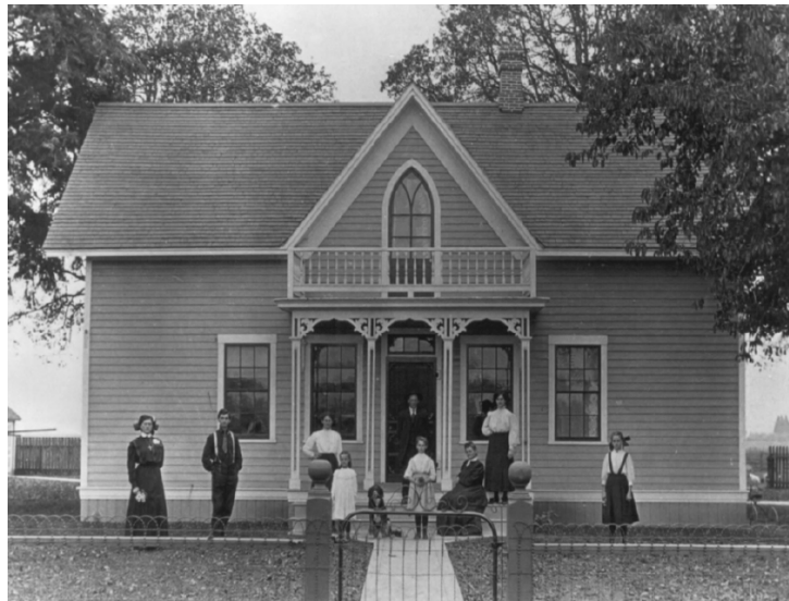
Figure 10. The Beeks house is a typical Gothic Revival house with cross-gabled roof and decorative porch. Bernard Family c. 1910. National Register of Historic Places: Beeks House.
