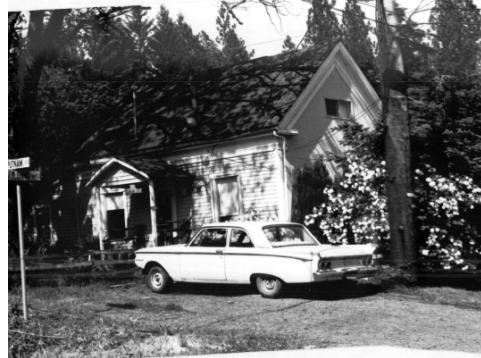
Worsley House 503 Spalding Ave Photo by Linn Co Inventory
